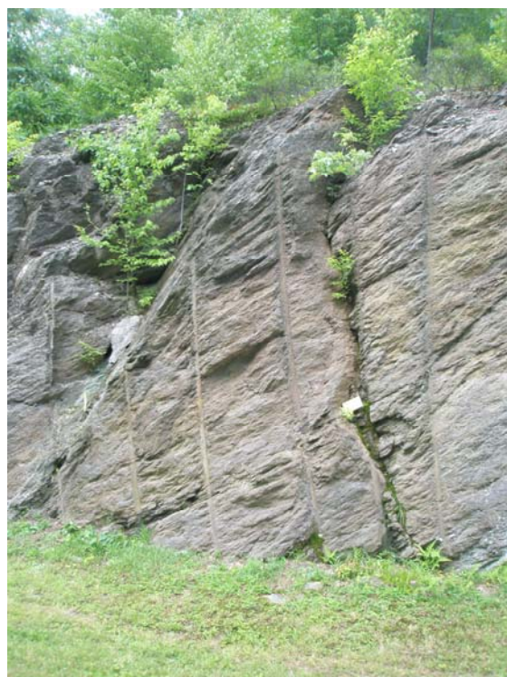
Fig. Stop 4A.1. A distant view of two Mesozoic faults: one dipping to the right (E) marked by the 20 cm long yellow notebook, and the other fault dipping to the left (W) with slickensides suggesting left-lateral motion.
