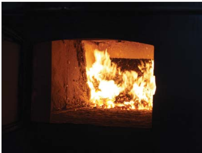
Firebox, showing burning wood chips, at Geremia Greenhouse in Wallingford.
