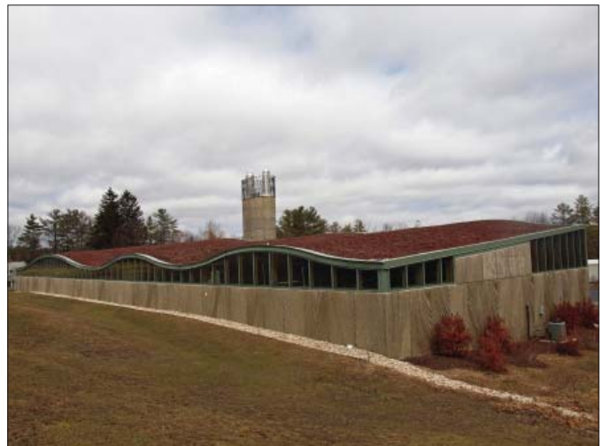
The central heating facility at Hotchkiss School. Seen in the picture is the building's green roof, one of many environmentally aware design decisions made in the construction of this building, leading it to be one of only 3 power plants nationwide to earn LEED recognition.
