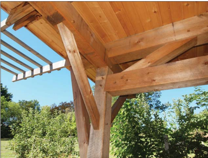
Native lumber used for structural purposes. According to the building code, these timbers must be assessed by a recognized grading agency.
