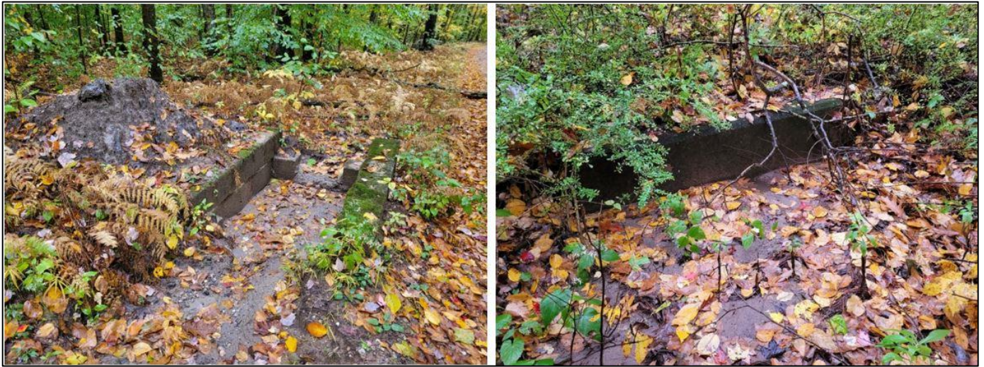
Photo 4.4. Photo to a culvert on Mulford Road, Mountain Block of Meshomasic State Forest. Both the inlet (left) and outlet (right) are filled in with sediment.
