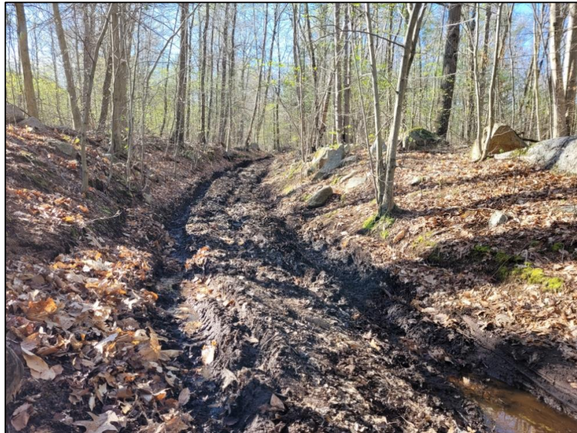
Photo 4.1. Photo of significant rutting and erosion caused by 4 x 4 truck and ATV usage on an abandoned town road within Meshomasic State Forest.
