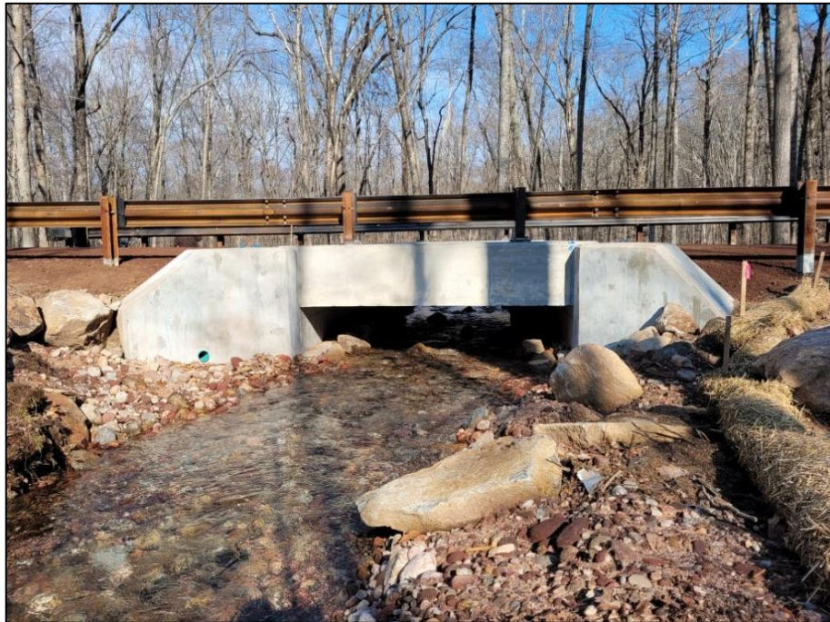
Photo 4.0. Photo of the completed Mott Hill Brook concrete, three-sided, bottomless box culvert. This new culvert, completed in January of 2023, conveys the Mott Hill Brook underneath Del Reeves Road.
