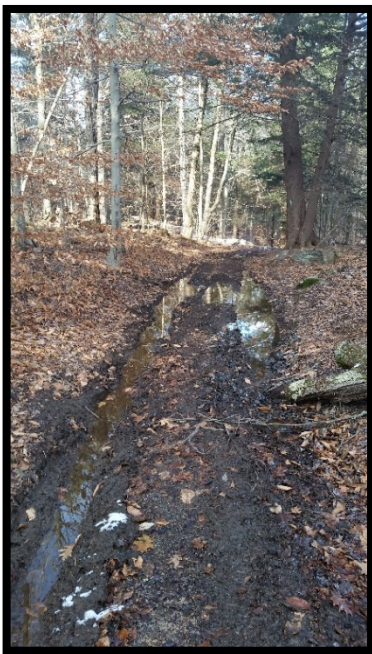
Figure 3. Old Town Road showing rutting from off-road vehicles.
