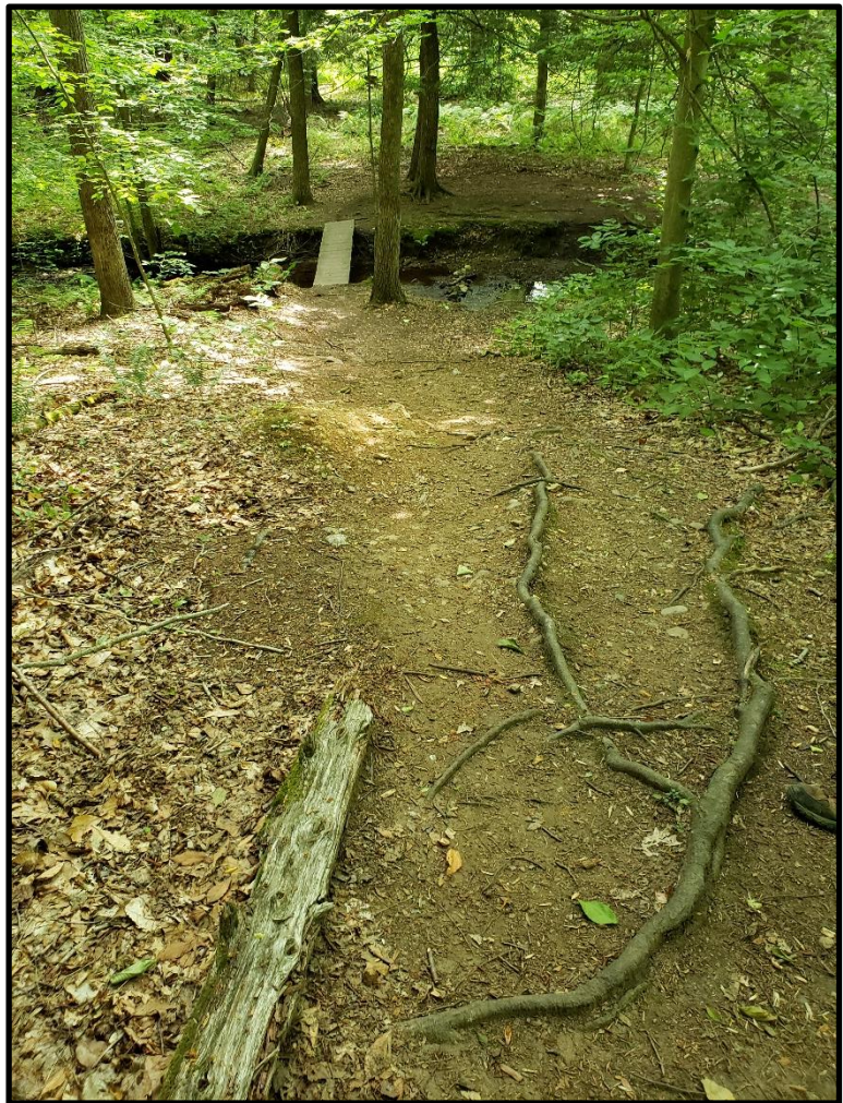
Figure 8. A heavily used spur trail in the Lower Block that is accessed from town property. The layer of organic matter has been removed, exposing mineral soil and roots. The sediment from this trail flows directly into the stream.
