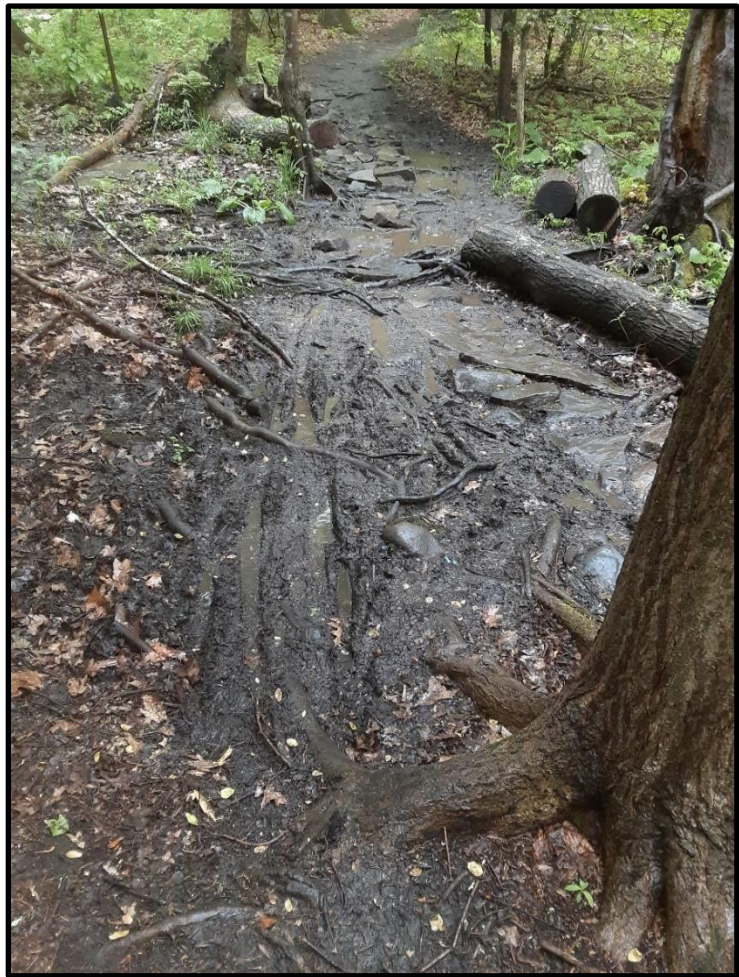
Figure 9. This trail is not part of the Blue-Trail system and is heavily used by both mountain bikers and hikers. When a trail crosses a wet area, it tends to widen as users try to find drier ground.
