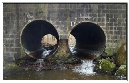
Figure 2. Example of culverts perched above streambed.
