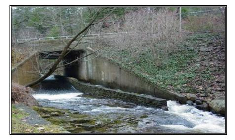
Figure 13. Example of fishway installed within a culvert.
