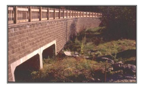
Figure 8. Example of vertical headwall that reduces length of culverts.
