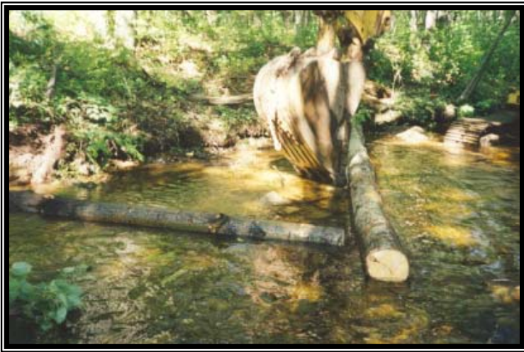
Installation of logs to create log/rock wing deflector.
