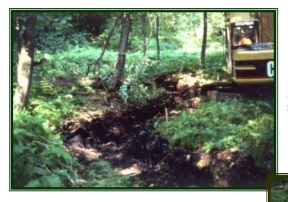
Rough-out excavation of new channel being relocated into wetlands.
