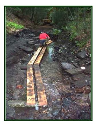
Installation of modified LUNKER, a fish habitat enhancement structure designed to create undercut bank habitats.
