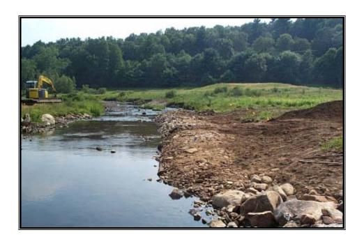
Photograph showing final grading, reduction in channel width and creation of bankfull bench.
