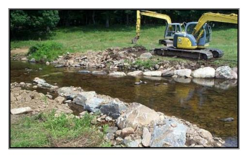
Completed construction of cross vane immediately below the upstream cattle crossing.
