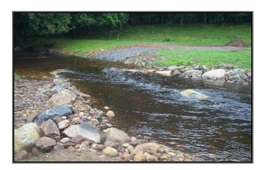
Photograph of cross vane during a storm event illustrating a primary function of the cross vane to redirect flow into the stream's centerline and away from the streambank.
