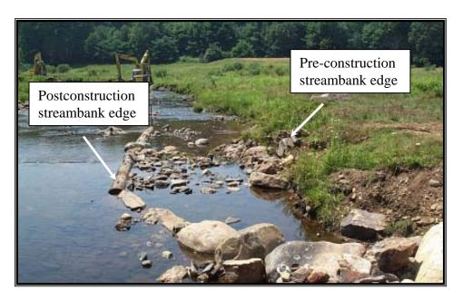
Photograph comparing preconstruction streambank edge and area of channel that will be filled to create the bankfull bench.
