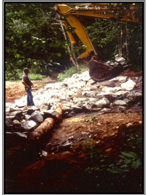
Installation of rock riprap over log core and across channel.
