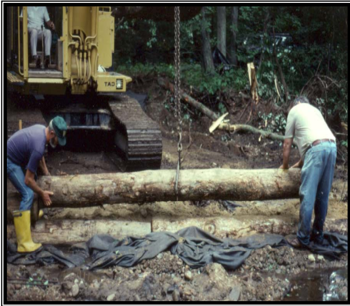
Installation of timber log core buried within channel block.
