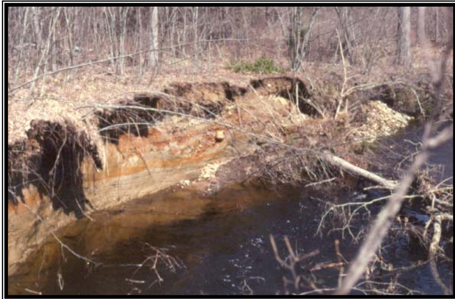
Meander bend bank erosion and instability in 1996 prior to restoration efforts.
