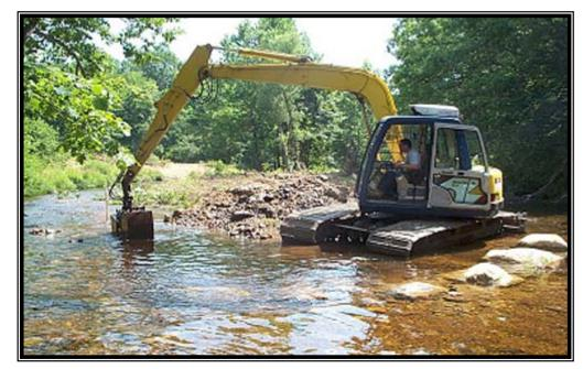
Construction of boulder J-Hook, a structure designed to redirect water away from streambank.
