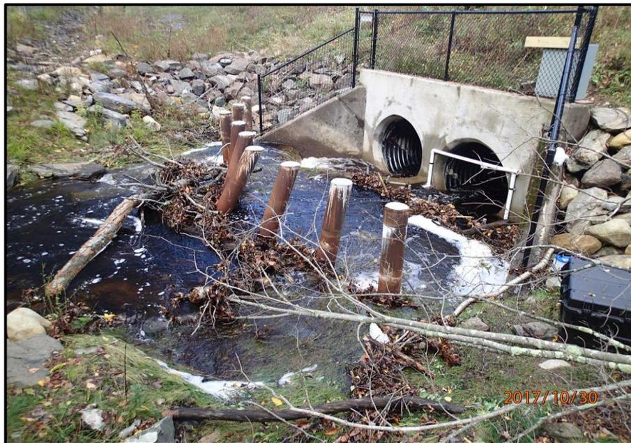
**Figure 6. View of secondary rebar trashrack and concrete diversion wall at inlet.**
