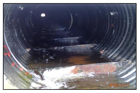
Figure 4. Upstream view of corner baffle system at moderate stream discharge.
