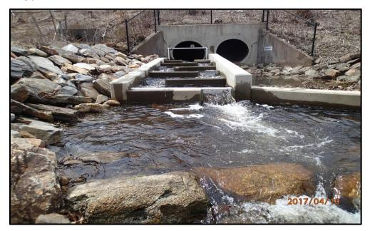
*Figure 3. Upstream view of concrete pool and weir fishway, diversion wall and boulder weir holding pool.*
