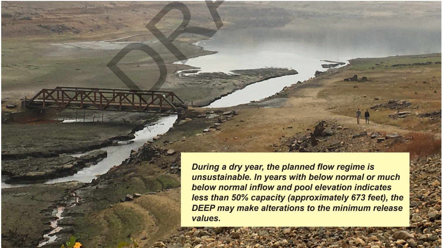
The northern portion of Colebrook River Lake during the fall of 2016. The entire flow of the West Branch of the Farmington River (15.9 CFS at the New Boston gage on 10/21/16 at 11:00 am) can be seen flowing under the Harvey Mountain Bridge and into the remaining Colebrook River Lake pool (elevation of 634.9 feet). The deck of the bridge is exposed when the lake is at 646.5 feet.
