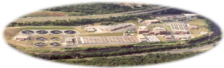
Waterbury Water Pollution Control Facility
