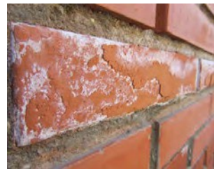
EFFLORESCENCE & SPALLING
