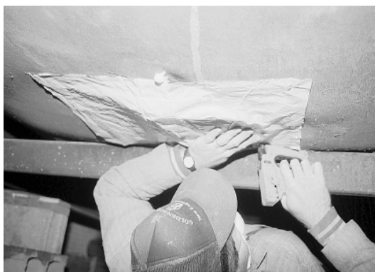
Blowing a floor through the belly: The contractor inserts a rigid fill-tube through the belly to blow insulation into the floor cavity and underbelly.
