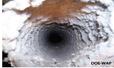
Lint collection: After years of operation, lint coats flexible pipe and eventually blocks the airway.
