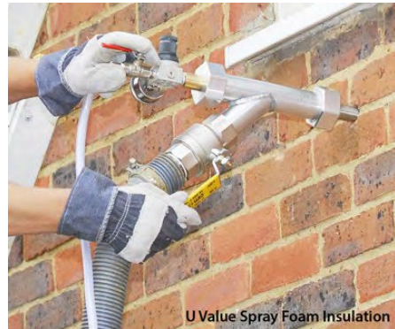
Injectable foam: Installers inject low-density foam into a cavity behind a single brick wall.
