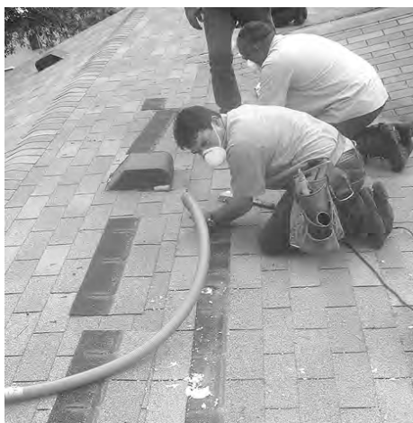
Blowing from the roof deck: Technicians remove a row of shingles, drill, and blow fiberglass into this vaulted roof cavity.
