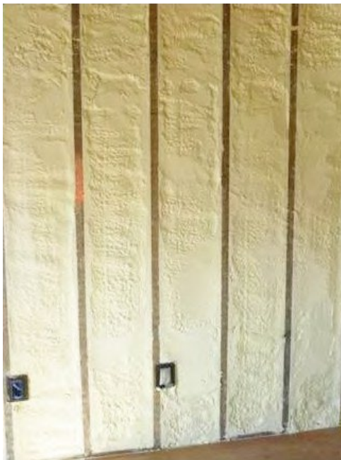
Sprayed closed-cell foam: Installers spray closed-cell foam short of filling the cavity or else they shave the excess off.
