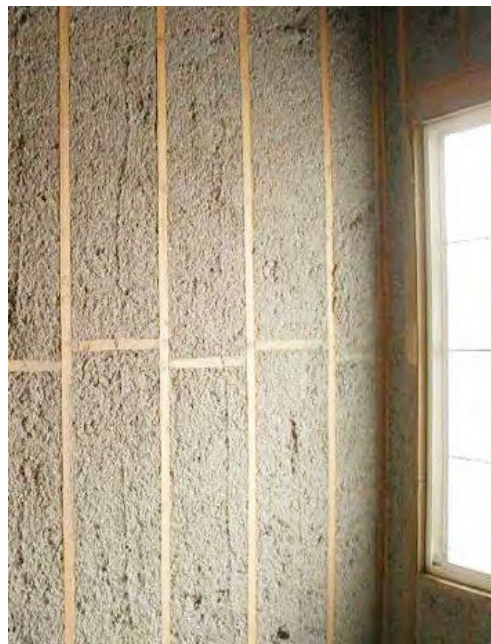
Spray fibrous insulation: Installers blow wet-spray fibrous insulation into cavities and shave off the excess.
