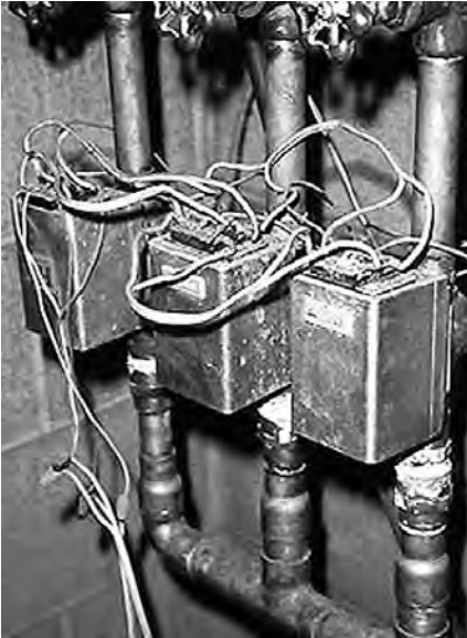
Zone valves: Separate thermostats control each zone valve. Zone valves have switches that activate the burner.
