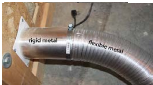
Vent and termination: Use rigid metal vent pipe if at all possible. Or use flexible metal vent and not foil vent when flexibility is required.
