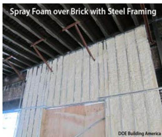
SPF insulates, seals, and reinforces brick wall: In this installation, open-cavity spray foam performs three separate functions.
