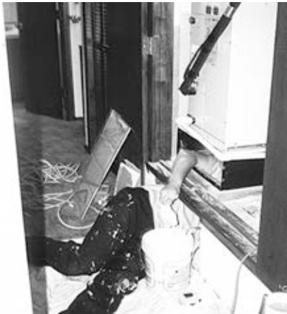
Lining a panned cavity: Foil-faced foam board, designed for lining cavities is sealed with duct mastic to provide an airtight return.
