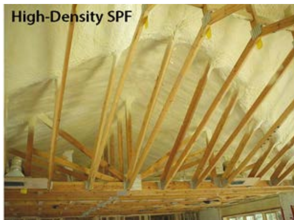
High density foam seals and insulates: High density foam can seal and insulate difficult areas in the same installation.
