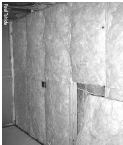
R-15 fiberglass batts: install unfaced batts as shown on the right. Cut the batts accurately and install them carefully.
