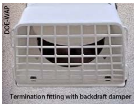
Vent and termination: Use rigid metal vent pipe if at all possible. Or use flexible metal vent and not foil vent when flexibility is required.
