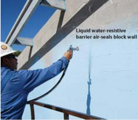
Liquid water-resistant barrier: This retrofit serves two purposes: water proofing and air sealing.
