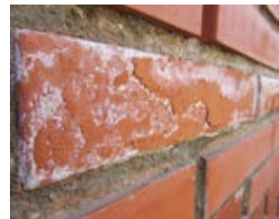
EFFLORESCENCE & SPALLING
