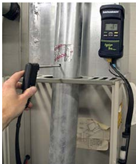
80+ Furnace: Measure draft and sample flue gases in the vent connector above the furnace.
