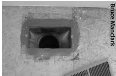
Sealing register boots: Seal between the boot and floor. Seal joints inside the boot.
