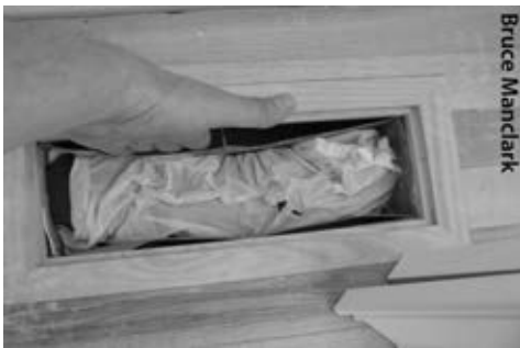
Sealing register boots: Seal between the boot and floor. Seal joints inside the boot.
