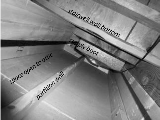
Stairway wall within the thermal boundary: Double wall forming the stairwell connects an unfinished area under the basement stairs with the living spaces, attic, and the space behind the finished basement walls.
