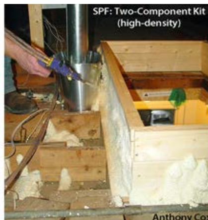
High density foam seals and insulates: High density foam can seal and insulate difficult areas in the same installation.
