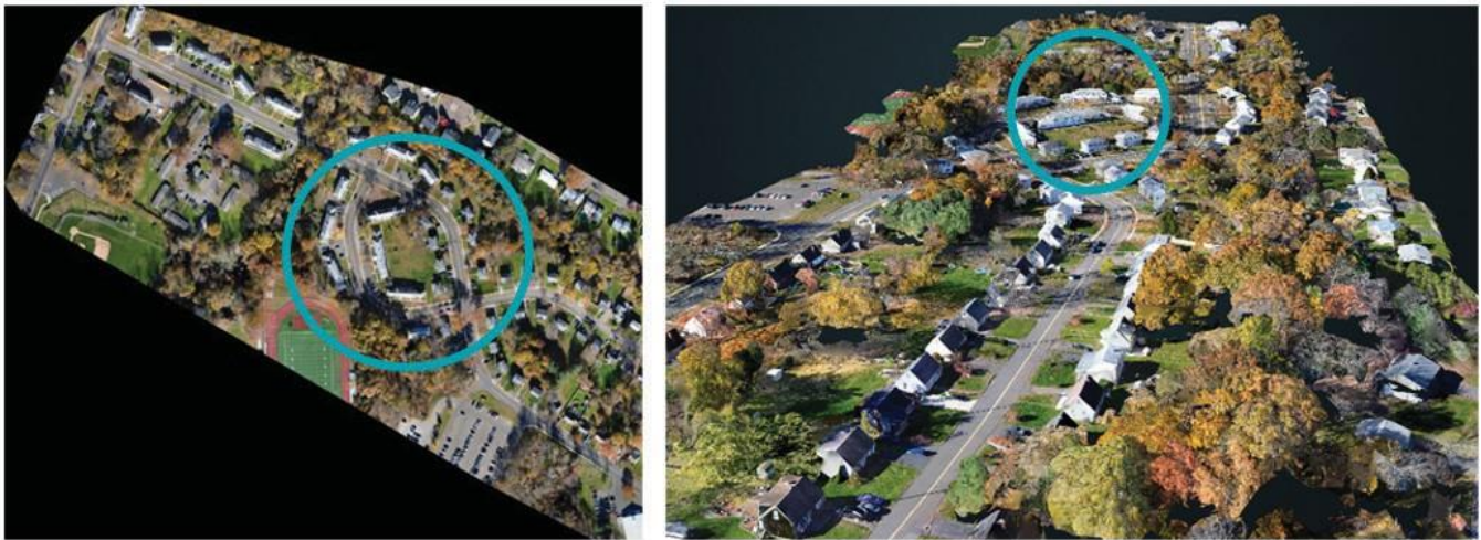
Figure 3. Aerial view of Ulbrich Heights with borefield location circled.
