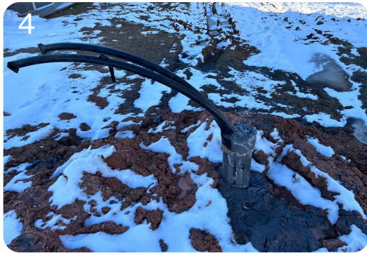
Borehole after grouting
