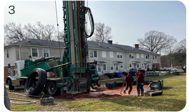
Drilling test borehole
