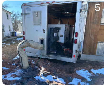
Insulated tubing and testing trailer
