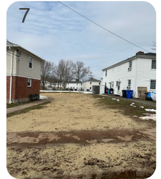
Borehole after cleanup
