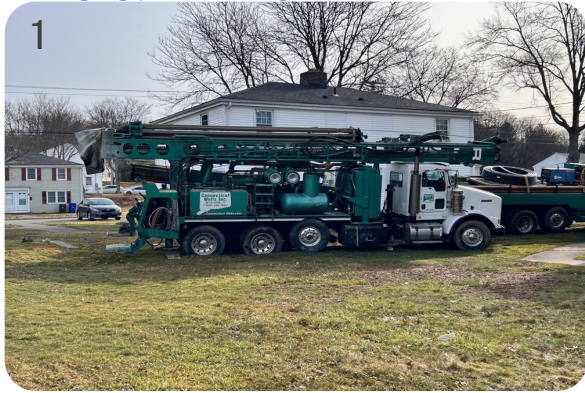
Drilling rig pre-levelling
