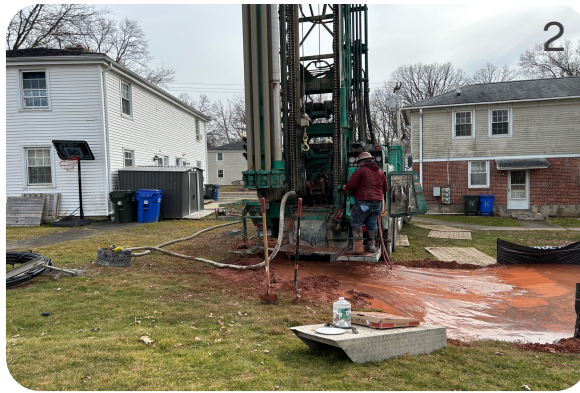
U-tube being put into borehole
