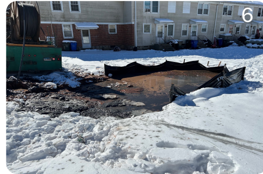
Drilling pond holding water and dirt
