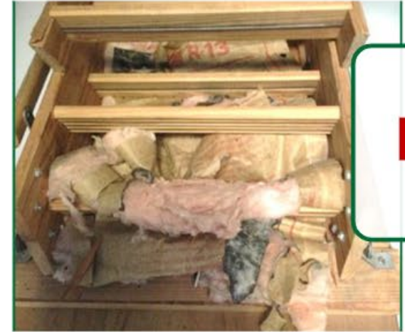
Sloppy Existing Insulation
