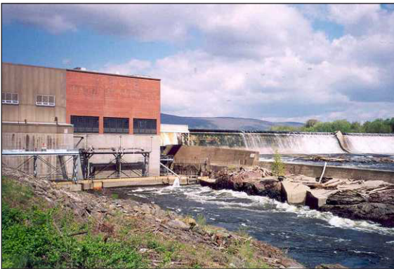
Holyoke Dam on the Connecticut River in Holyoke, MA
