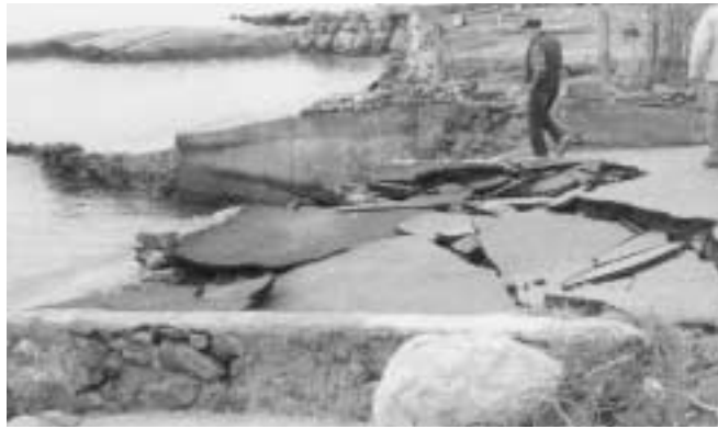
Inspectors assess damage to a seawall and pavement along Chapman Road, in Westbrook, caused by Storm Beth in 1992.
