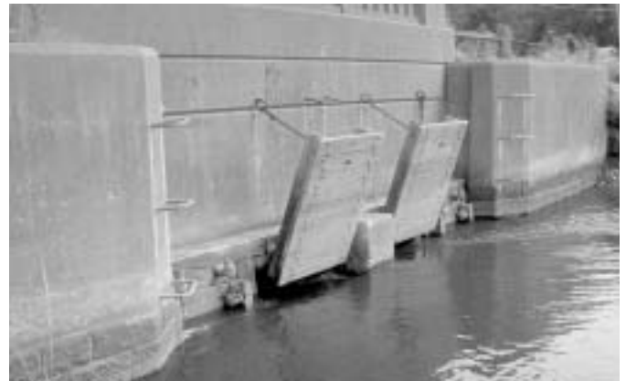
Tide gates, once used to drain a wetland, are managed (opened) to restore tidal flow to the extent necessary to restore an ecosystem.
