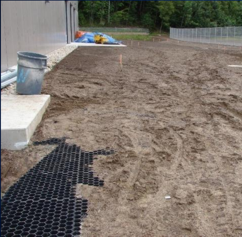
GrassPave Grid Stabilizes Un-Paved Delivery Entrance
