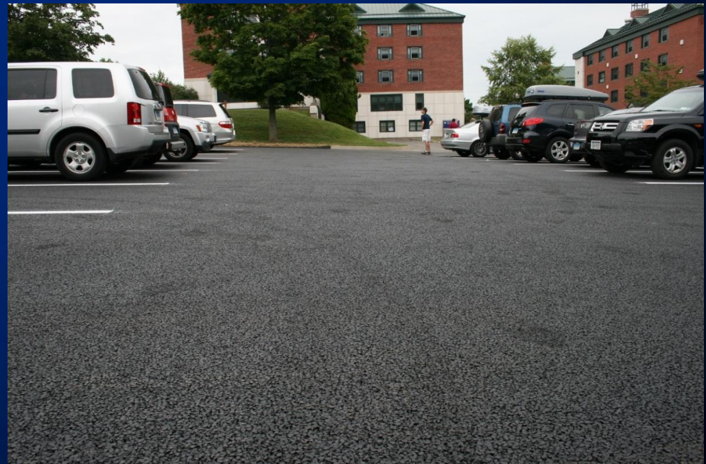
Permeable Asphalt Parking Lot Installed at Towers Residence Halls
