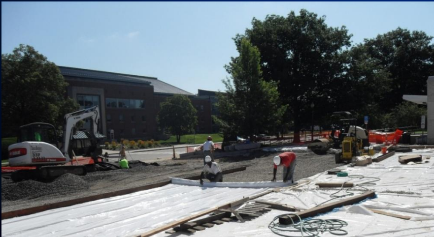
Workers Installing Porous Concrete Parking Lot at Greer Field House
