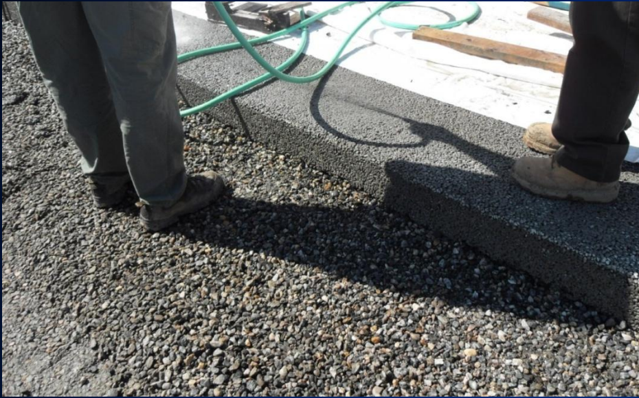
Workers Installing Porous Concrete Parking Lot at Greer Field House
