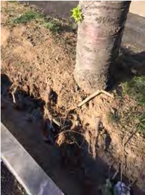
Roots chopped for granite curb installation
