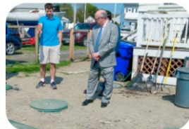
Residential septic and sewer tie-in
