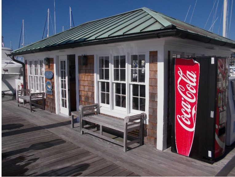
Existing Fuel Hut and Dock Marina Office
