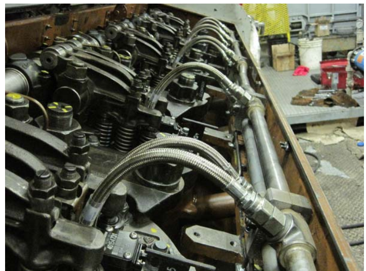
Fuel lines and jumpers installed
