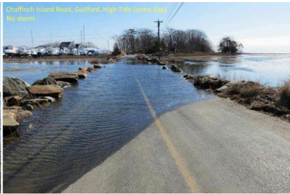
Frequent, tide-generated "nuisance" or "sunny-day" flooding on Chaffinch Island Road, Guilford was alleviated by elevating the roadway Photo Credit: Joel Stocker
