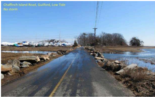
Frequent, tide-generated "nuisance" or "sunny-day" flooding on Chaffinch Island Road, Guilford was alleviated by elevating the roadway Photo Credit: Joel Stocker
