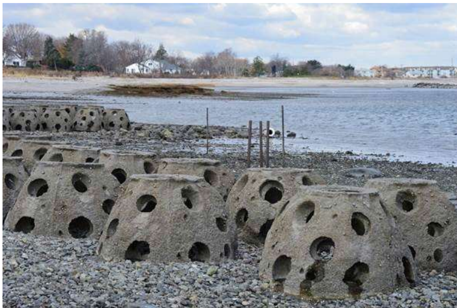
Installation of a reef ball living shoreline, Stratford Photo Credit: CT DEEP
