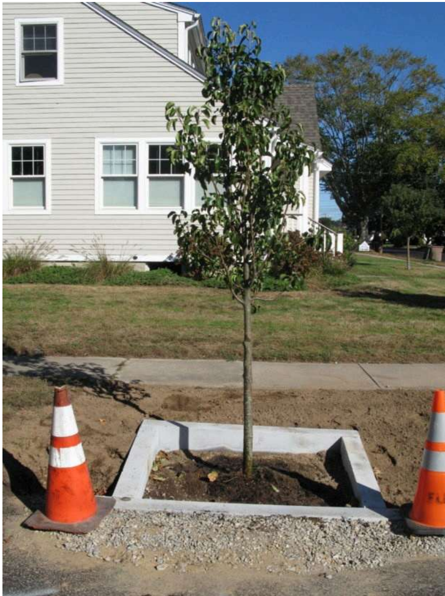
A "tree well" treats stormwater in East Lyme Photo Credit: Judy Rondeau, Niantic River Watershed Coordinator
