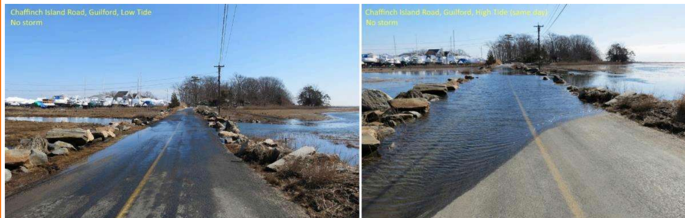
Frequent tide-generated "nuisance" or "sunny-day" flooding on Chaffinch Island Road, Guilford which has been alleviated by elevating the roadway
