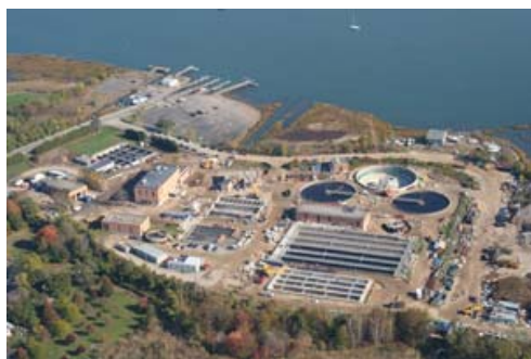
Stratford, Connecticut STP near Long Island Sound View Larger Image
