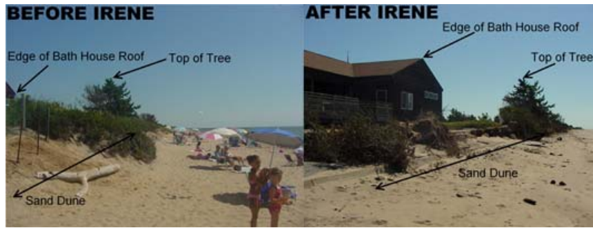
Damage to Dune at Hammonasset Beach State Park after Tropical Storm Irene View Larger Images
