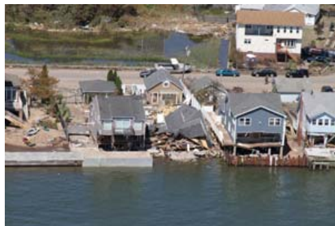
Damage from Tropical Storm Irene on Cosey Beach Avenue, East Haven View Larger Image
