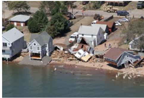
Tropical Storm Irene caused significant damage at Cosey Beach, East Haven View Larger Image
