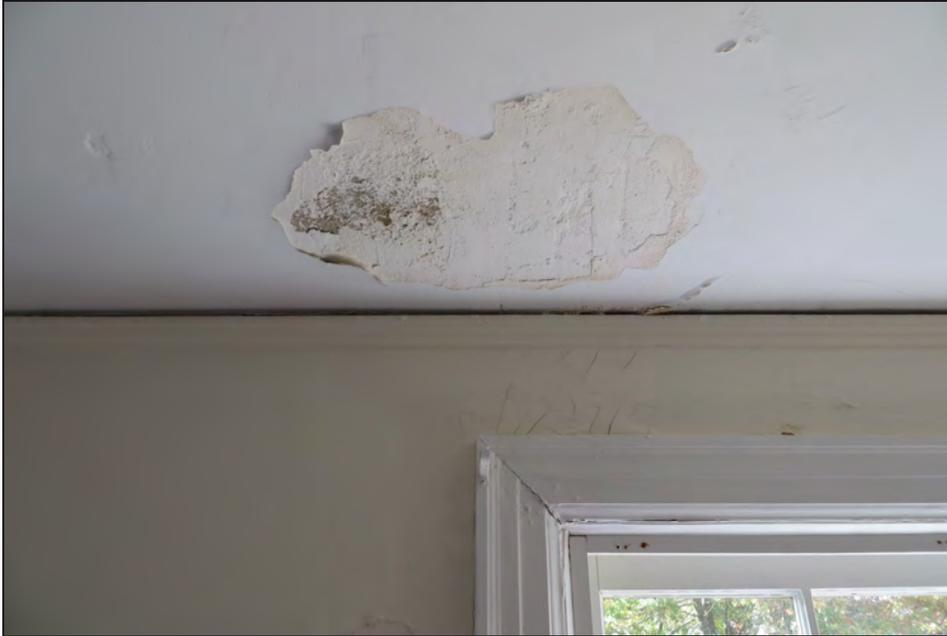
*After Superstorm Sandy damaged the roof of a historic house in Greenwich, water infiltrated the building. Left unattended, such damage can lead to mold or even weaken the structure. Credit: Greenwich Historical Society.*
