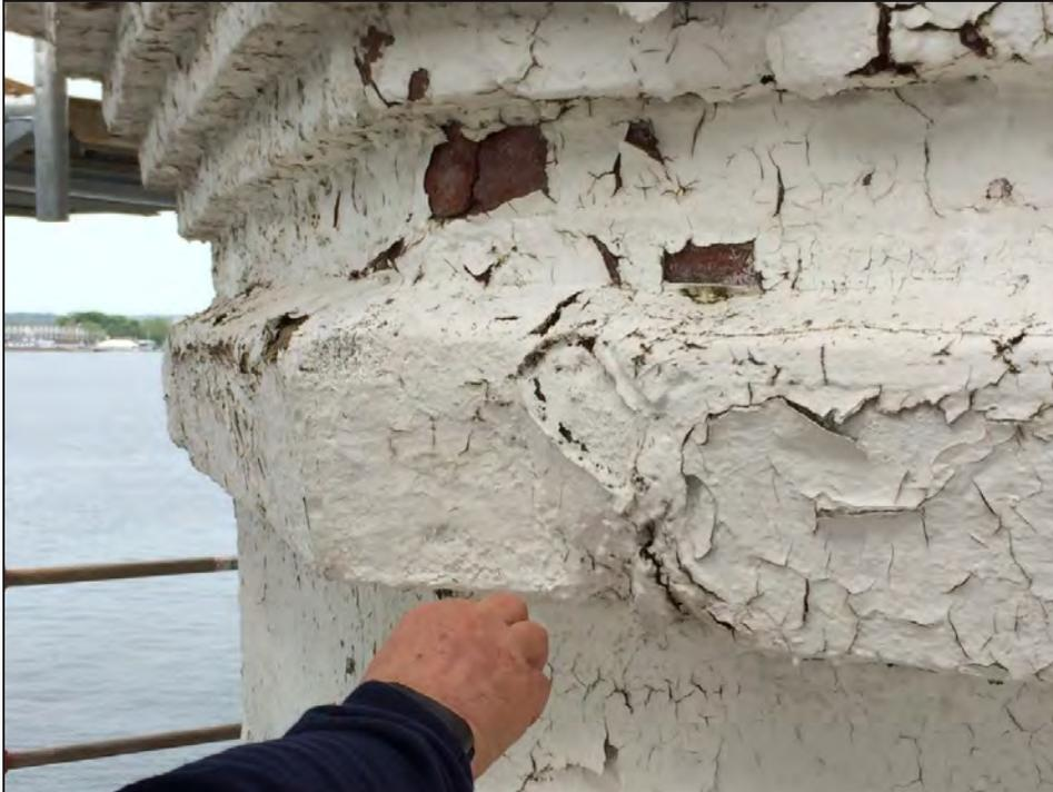
*Blistering or peeling paint, as at the Fayerweather Lighthouse in Bridgeport (1823, NR), indicates trapped moisture—in this case, at least partly the result of infiltration from a cracked lantern slab atop the brick corbelling. Credit: Douglas Royalty/SHPO.*
