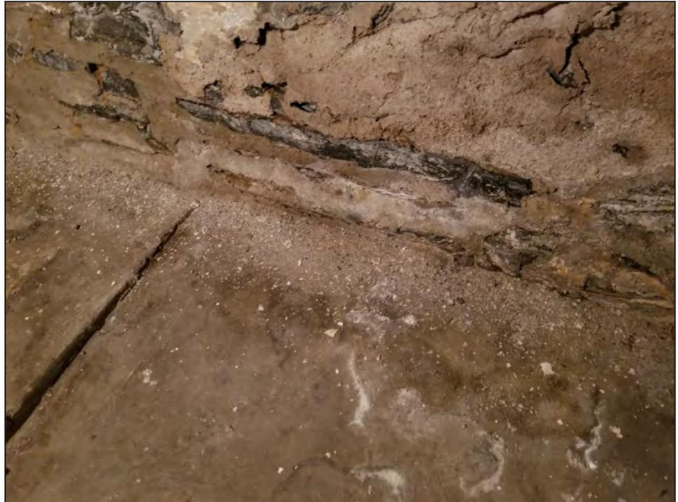
*Repeated water infiltration can erode lime mortars and deposit salts during evaporation. Credit: RCG&A.*
