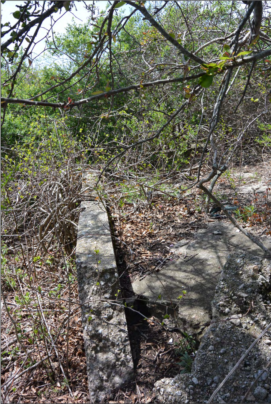
Poured concrete foundation and floor of structure on Pine Island (Photo by R. Christopher Goodwin & Associates)
