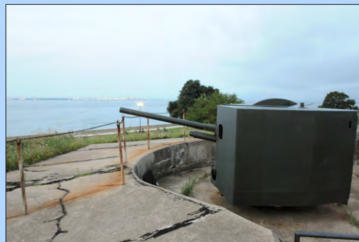
The two fixed-mount 90mm guns installed as part of the Anti Motor Torpedo Boat Battery (AMTB-915) on Pine Island during World War II looked like this gun installed on Battery Parrott, at Fort Monroe, Va. (photo by Neal Snyder, U.S. Army Environmental Command)
