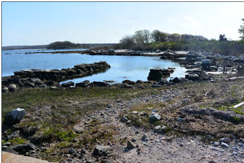
Photograph of the boat slip showing the retaining wall and wood pilings along the shoreline. Brick and other debris on the beach in the foreground are probably remnants of the fish processing plant and AMTB-915 activity (Photo by R. Christopher Goodwin & Associates)
