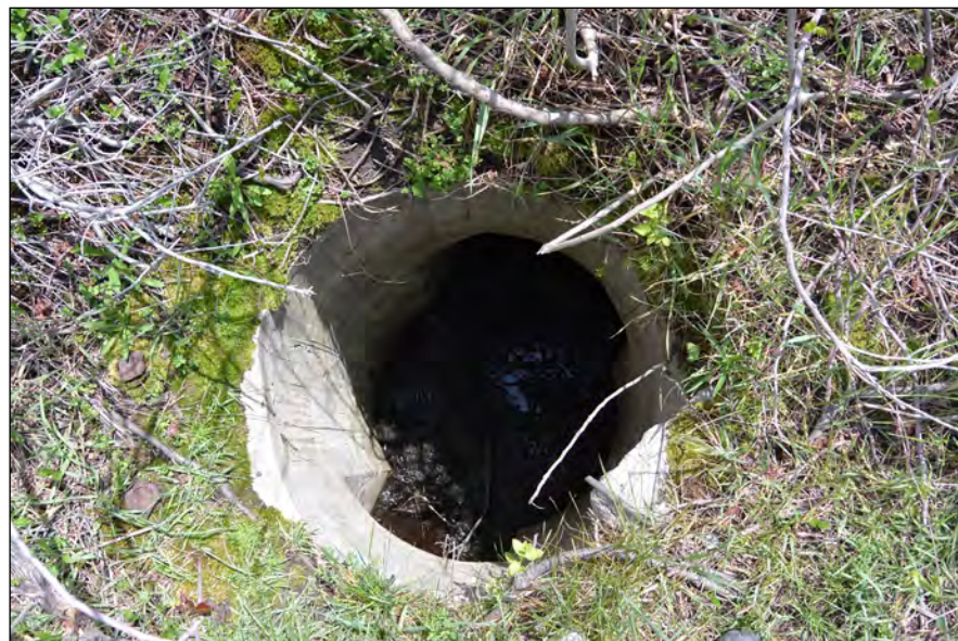
Photograph of concrete tunnel beneath the gun mount in the firing platform for one of the 90-mm guns at AMTB-915 on Pine Island (Photo by R. Christopher Goodwin & Associates)
