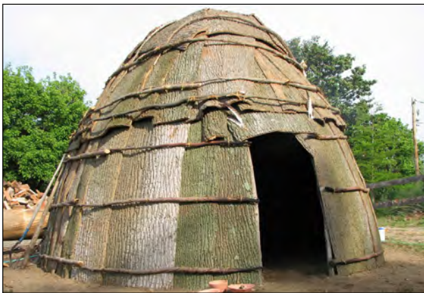
The Quinnipiac people lived in wigwams, a common house type among Native Americans in New England (Photo: Lost Towns Project, Inc.)
