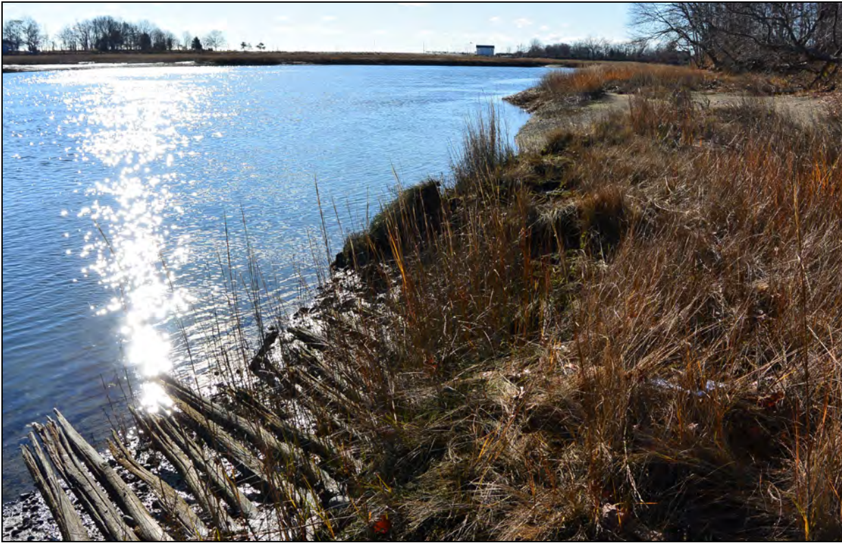
Log “punchings” of the corduroy road eroding from the bank of Ash Creek with Great Marsh Island in the distance (Photo by R. Christopher Goodwin & Associates, Inc.)
