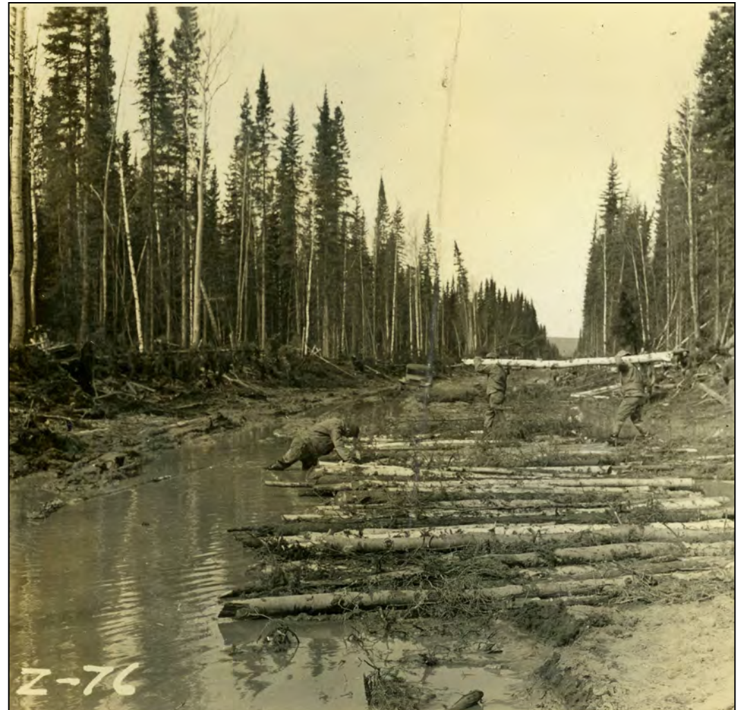
Building a corduroy road as part of the Alaska-Canada Highway ca. 1942 (Source: photograph possibly by Staff Sargent R. Schubert, courtesy of Office of History, Headquarters, U.S. Army Corps of Engineers, Alexandria, Va.)
