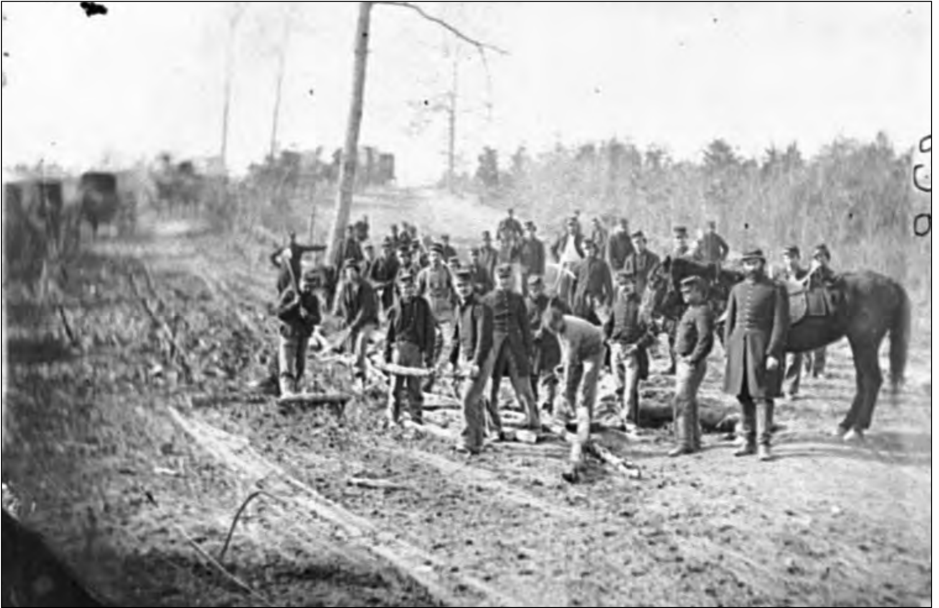
Building a corduroy road near Richmond, Virginia, in June 1862 (photograph by David B. Woodbury; Source: Library of Congress)
