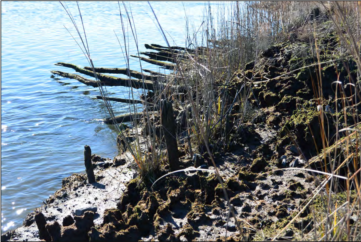
Photo of logs of the corduroy road eroding from the bank of Ash Creek with stabilizing stakes visible (Photo by R. Christopher Goodwin & Associates, Inc.)
