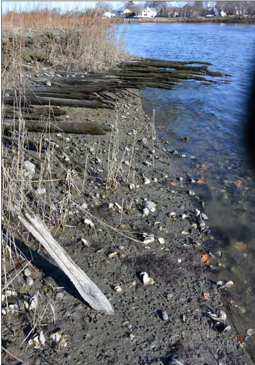
Logs of the corduroy road eroding from the bank of Ash Creek (Photo by R. Christopher Goodwin & Associates, Inc.)
