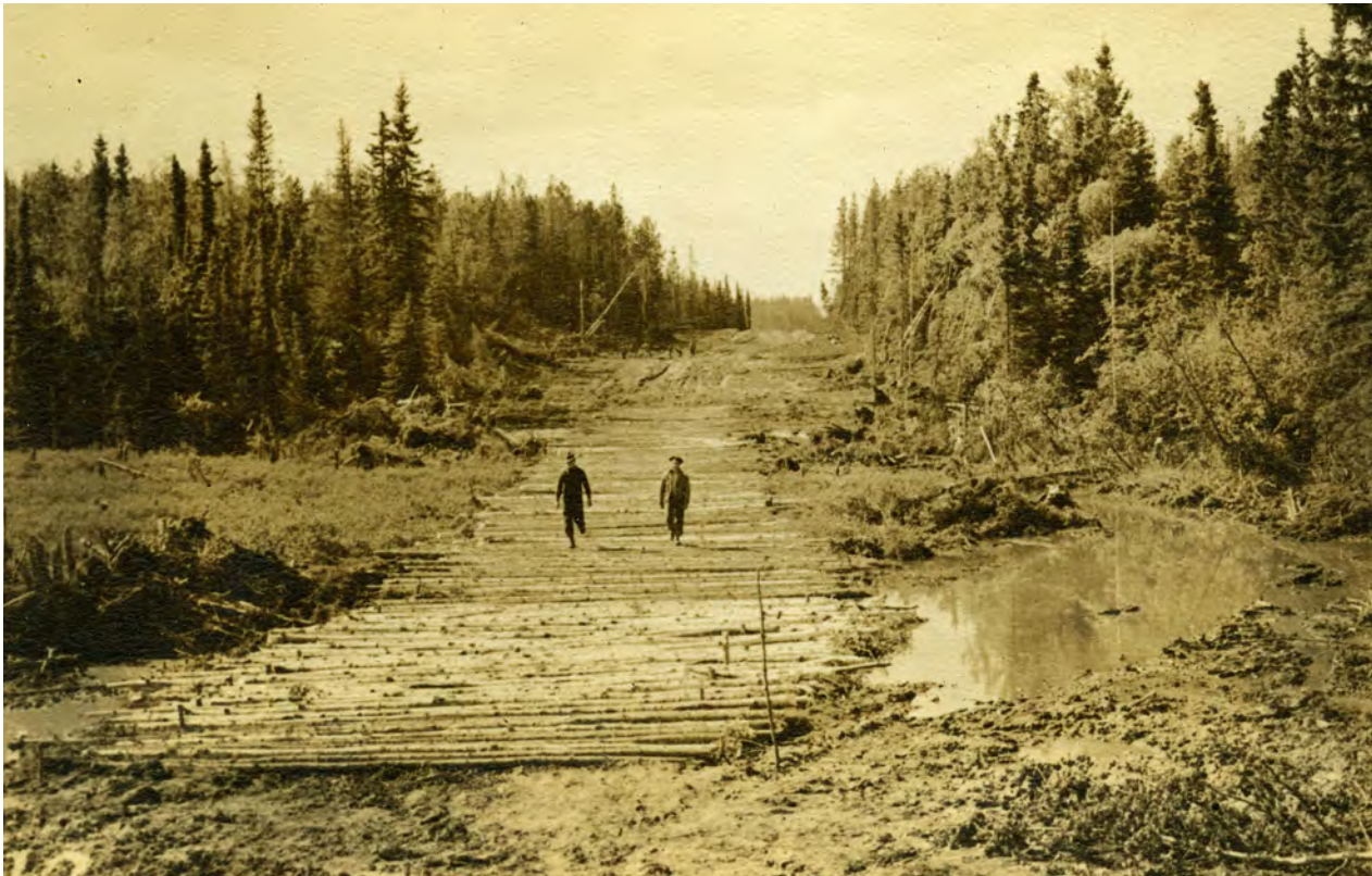
Colonists and early Americans built corduroy roads to negotiate soggy low-lying terrain (Photograph from the Alaska Highway Scrapbook ca. 1942-3; Office of History, Headquarters, U.S. Army Corps of Engineers, Alexandria, Va.)
