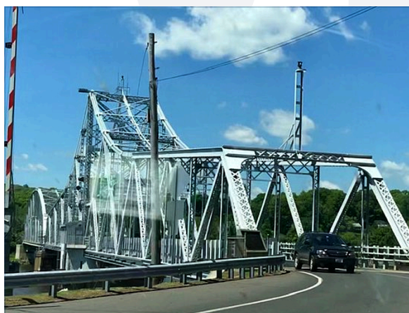
— East Haddam Swing Bridge, Haddam, CT.
