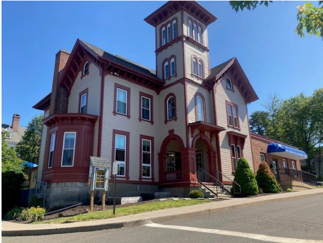
Municipally owned building by the City of Bristol- 51 High Street. Exterior carpentry repairs and painting.
