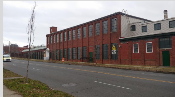
Hartford Special Machinery Company Complex, 287 and 296 Homestead Ave., Hartford
