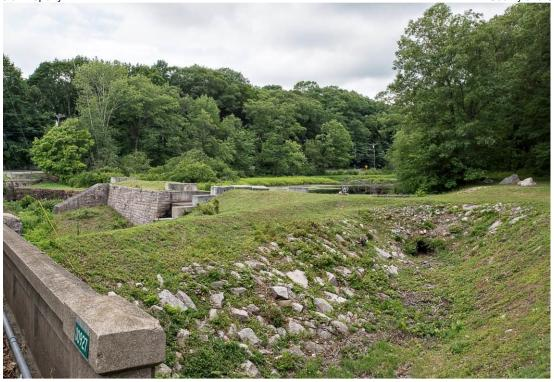
Photo 34. View south from Route 32 bridge showing dam, Picker Pond and abandoned head race.
