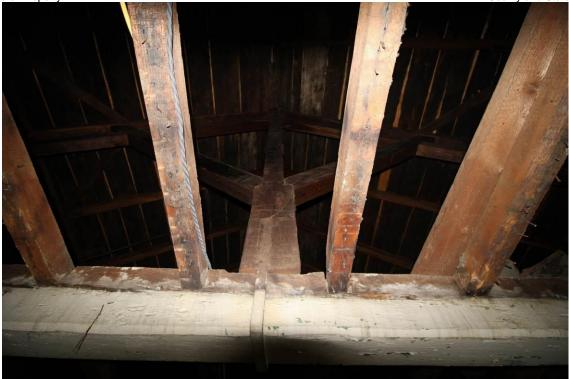
Photo 11. Interior of the top floor of Building M-4A looking to the kingpost roof truss.
