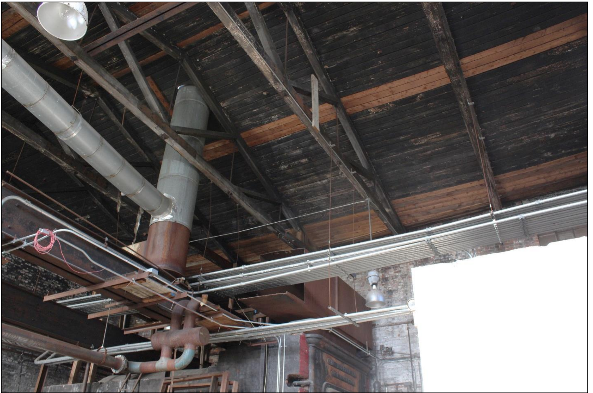
Interior roof structure of Building No.2 (1919), camera facing northeast. Photograph 16 of 27
