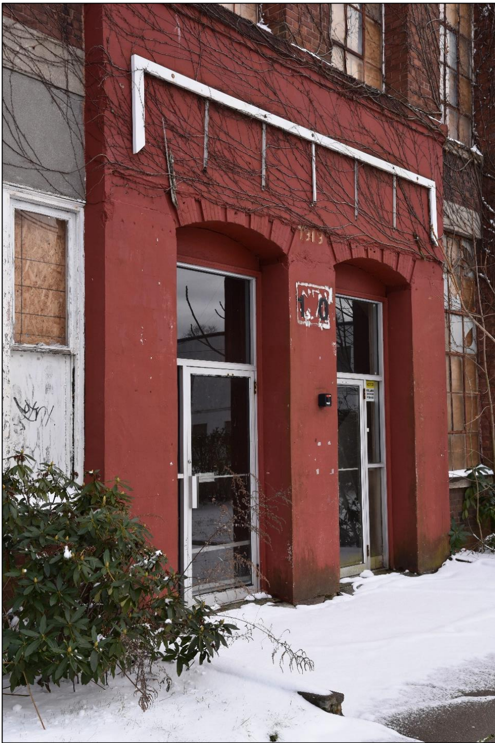
Detail of portico on Building No. 1 (1919), camera facing southwest. Photograph 3 of 27
