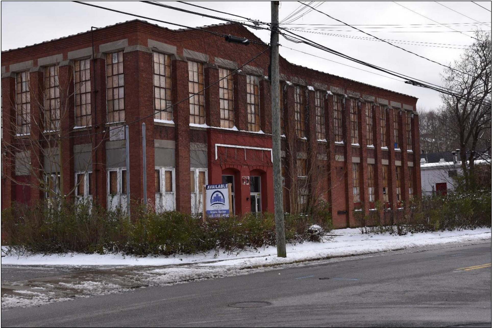
North elevation (façade) of Building No. 1 (1919), camera facing southwest. Photograph 2 of 27
