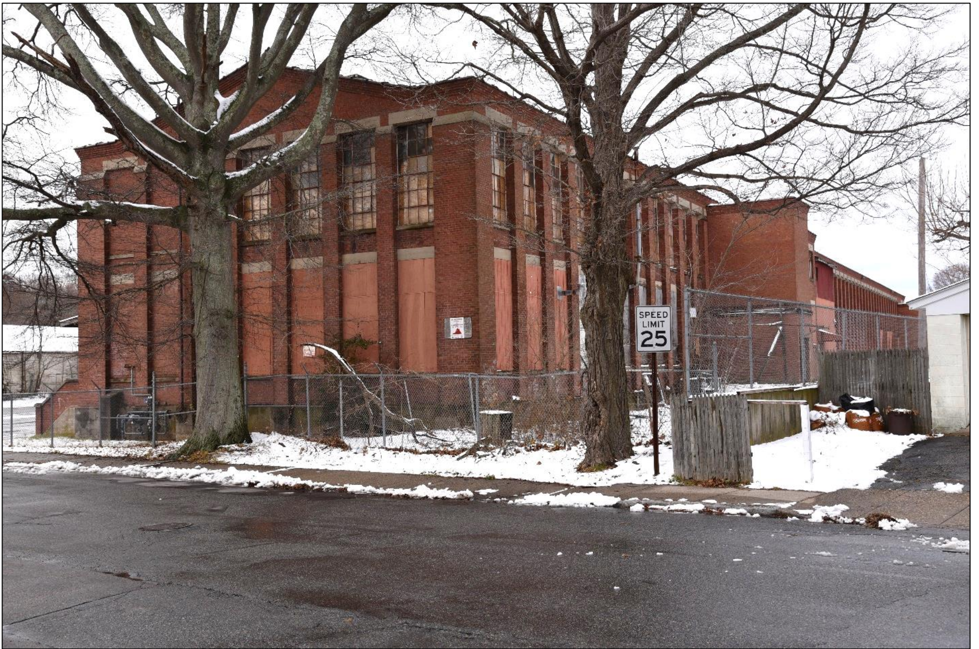
Southern and western elevations of Building No. 3 (1922), camera facing northwest. Photograph 22 of 27
