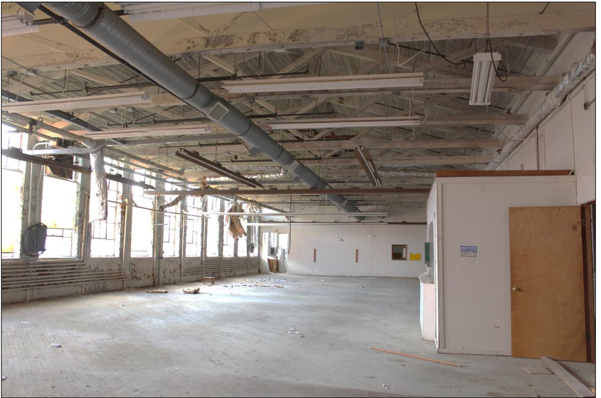
Interior second floor of Building No. 1 (1919), camera facing southwest. Photograph 10 of 27
