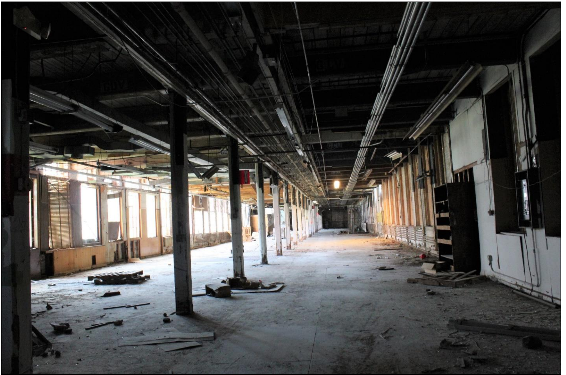
Interior first floor of Building No. 1 (1919), camera facing southwest. Photograph 9 of 27
