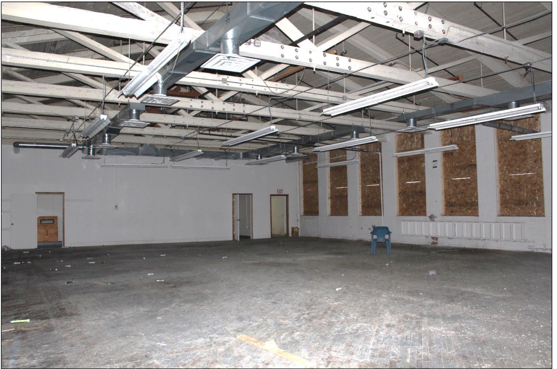
Interior second floor of Building No. 1 (1919), camera facing northeast. Photograph 11 of 27
