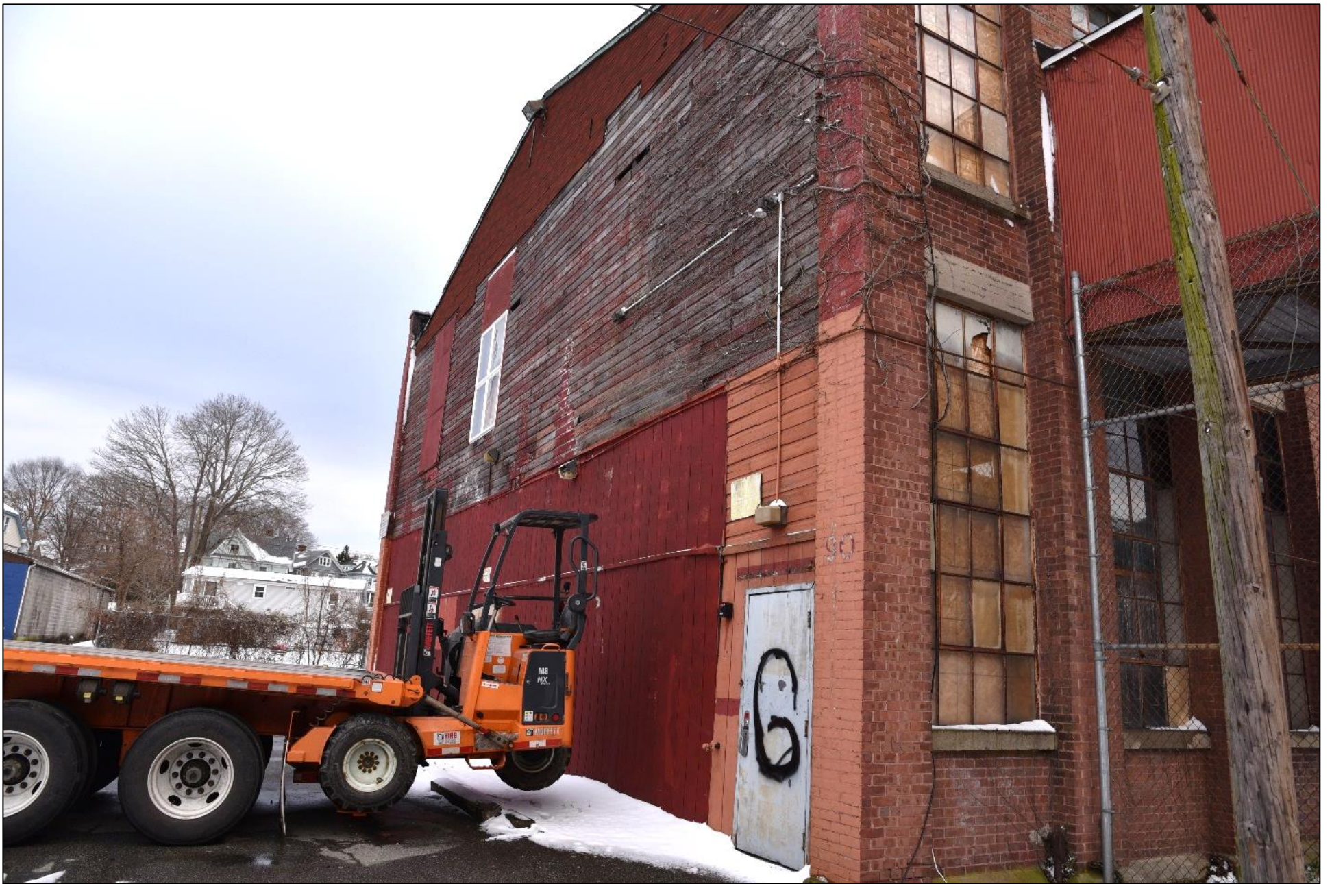
Detail of northern elevation of Building No. 3 (1922), camera southeast. Photograph 21 of 27
