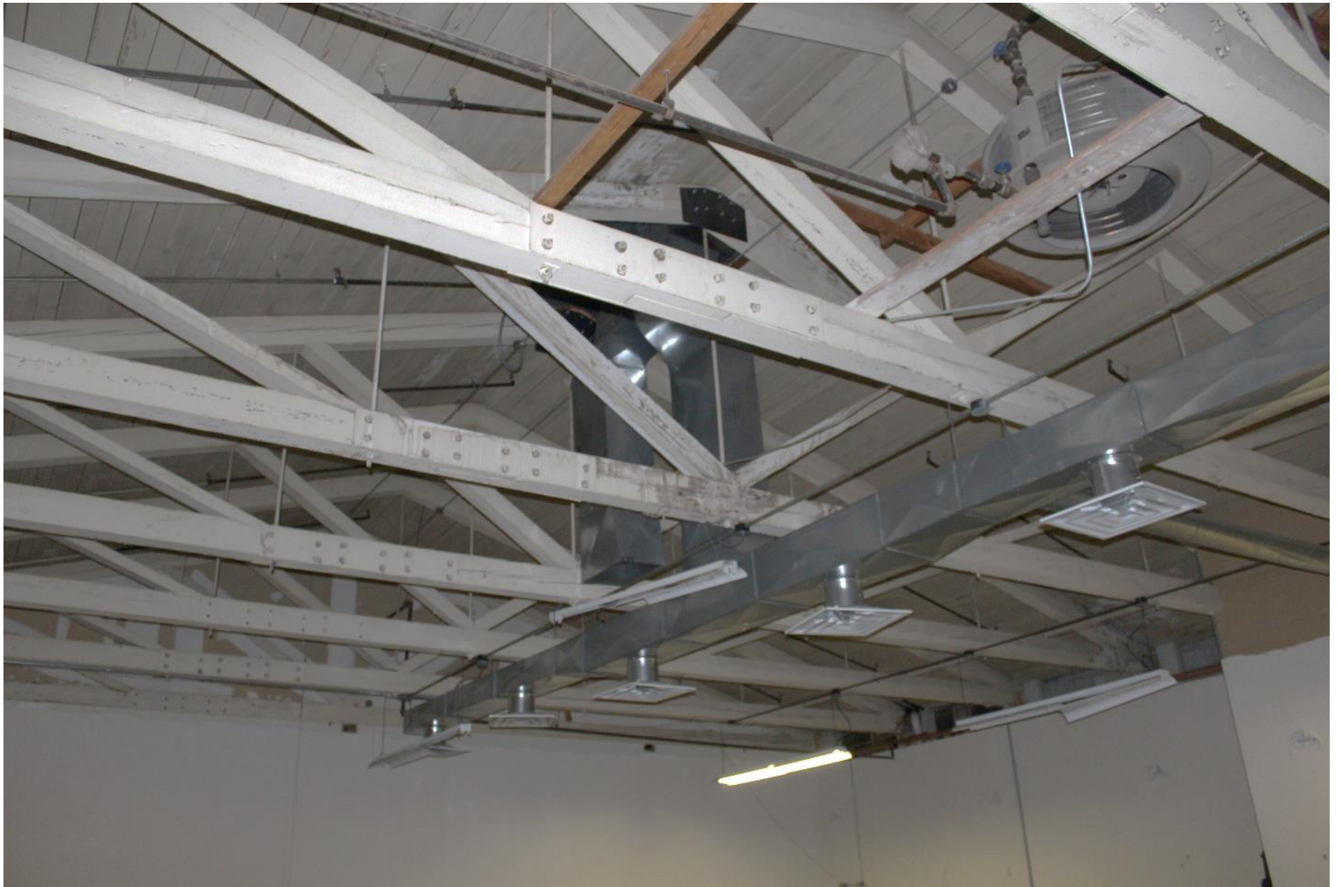
Interior second floor of Building No. 3 (1922), camera facing northeast. Photograph 27 of 27
