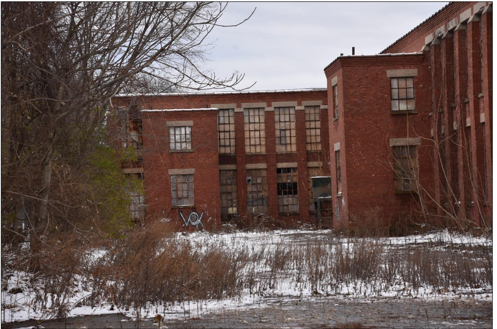
Southern Elevation of Building No. 1 Ell (1919), camera facing north. Photograph 7 of 27
