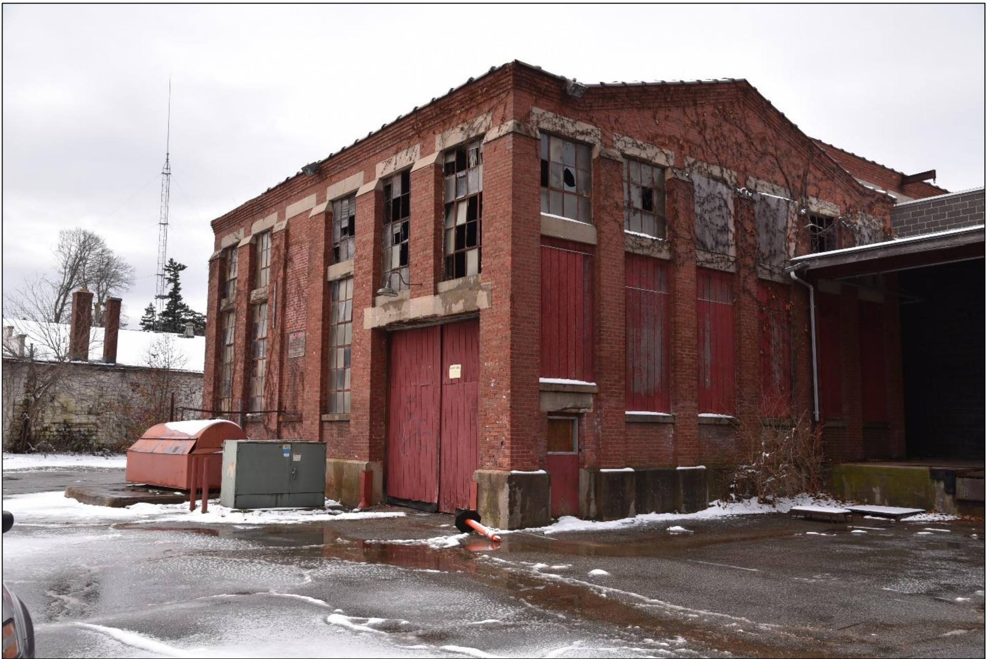
Southern and eastern elevations of Building No. 2 (1919), camera facing northwest. Photograph 15 of 27
