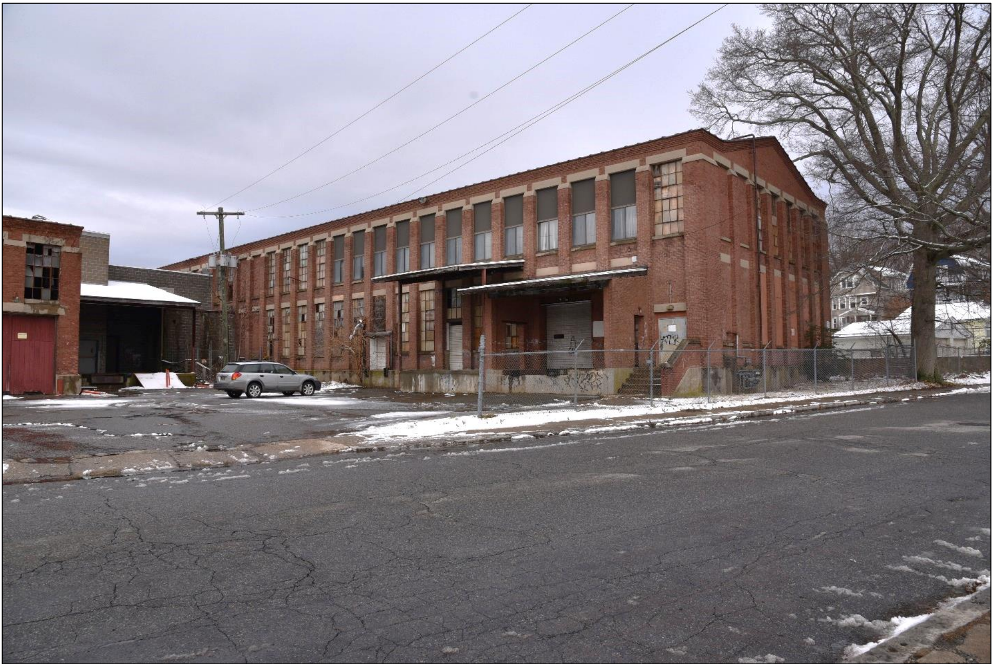
Eastern and southern elevations of Building No. 3 (1922), camera facing northeast. Photograph 23 of 27
