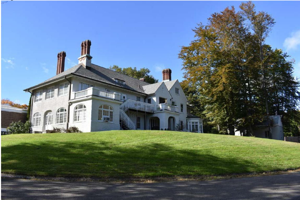
Photograph 18. Gray Gables (left) and Garage (right), looking northwest.
