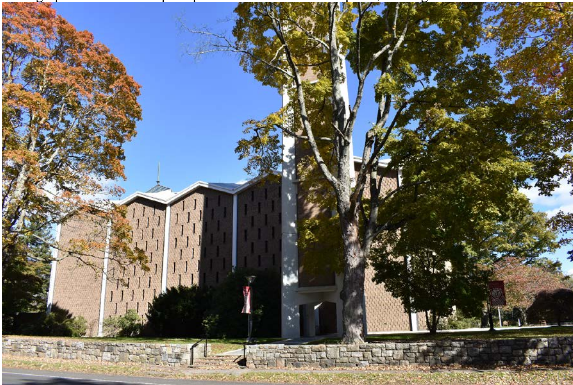
Photograph 4. St. Mark's Episcopal Church west elevation, campanile tower, and stone boundary wall, looking east.
