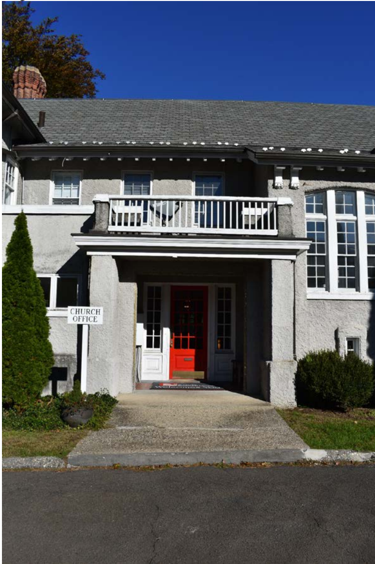
Photograph 17. Gray Gables entrance, looking east.
