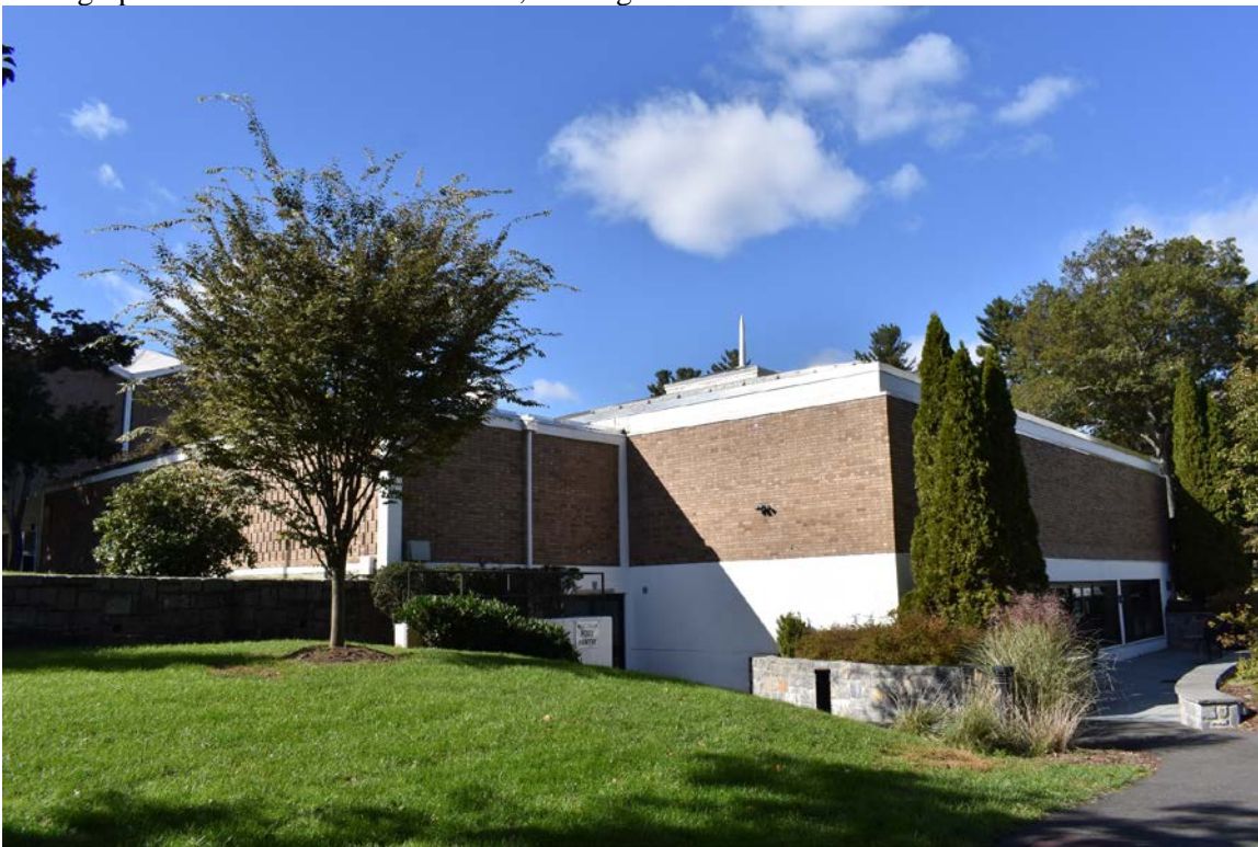
Photograph 11. Morrill Hall and entrance to lower teen room, looking northwest.
