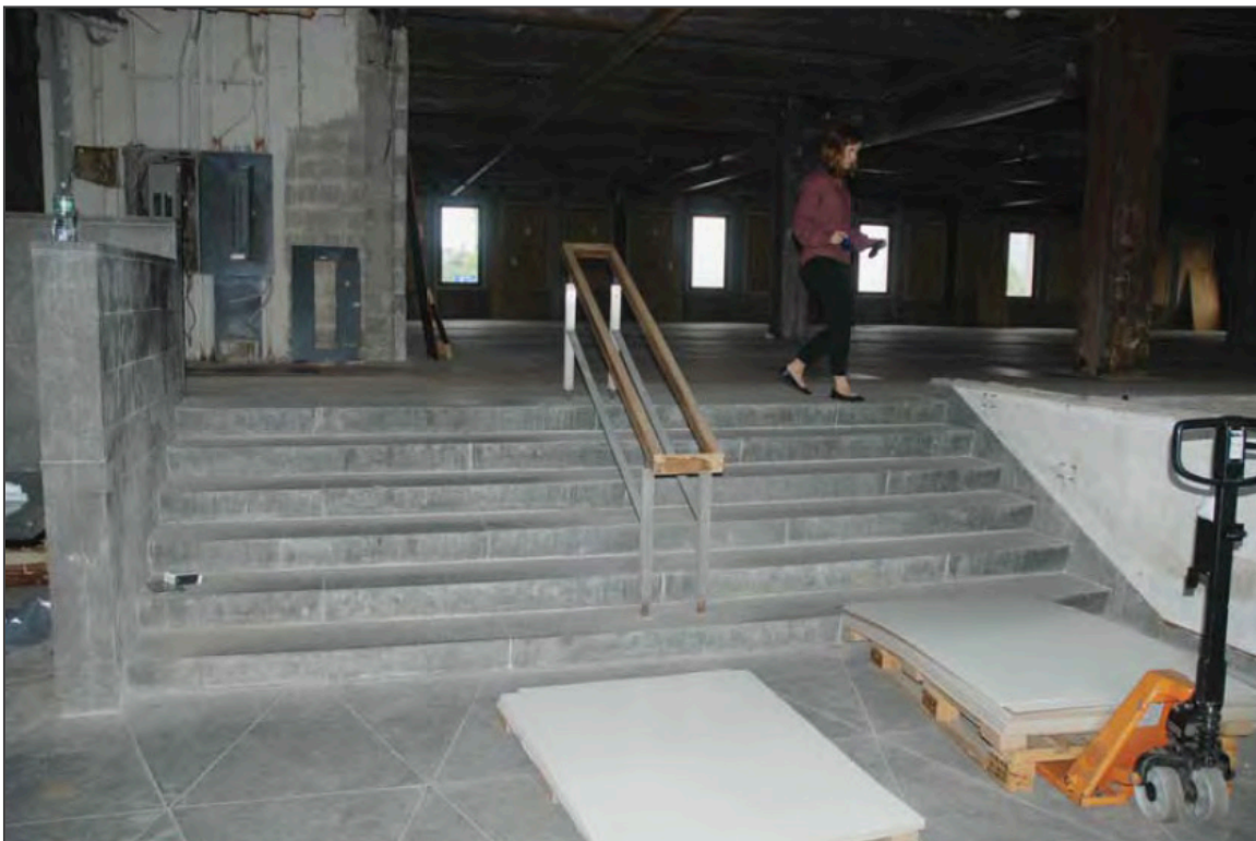
10. First floor lobby stair
