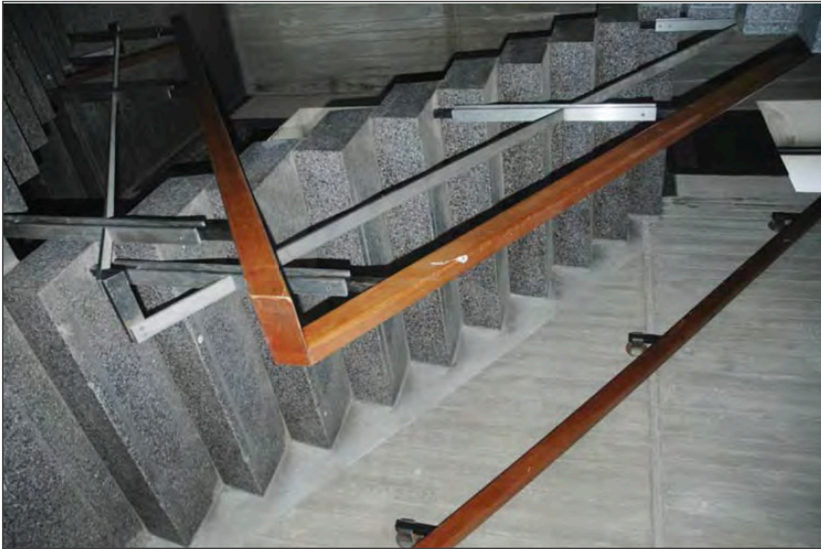
19. Seventh floor, main stair landing
