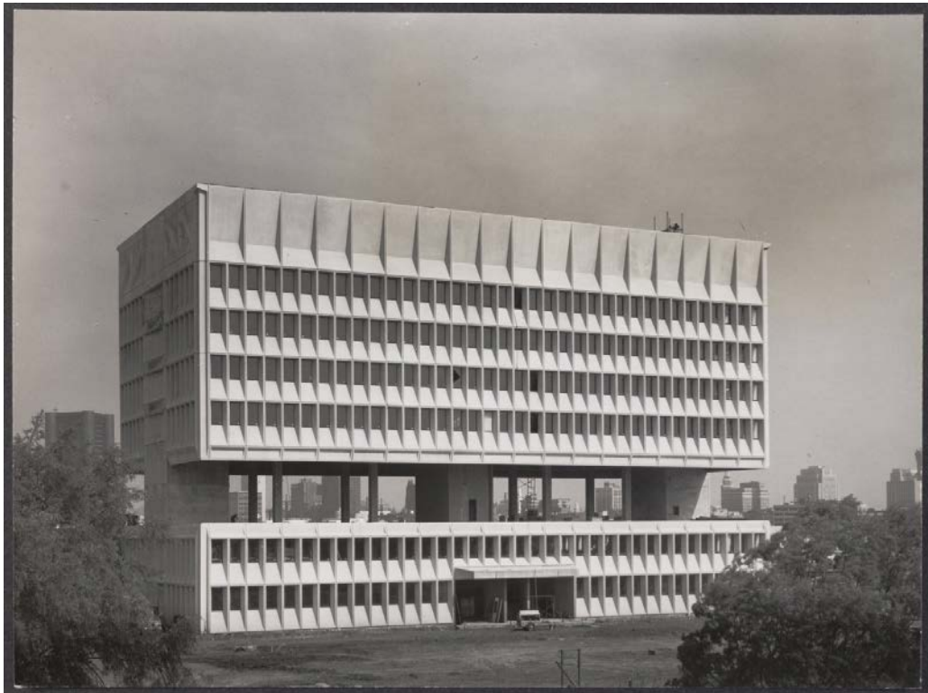
Figure 6: Construction photograph of the Armstrong Rubber Company Building, view towards east elevation, 1969 (Source: Syracuse University Libraries 2018)
