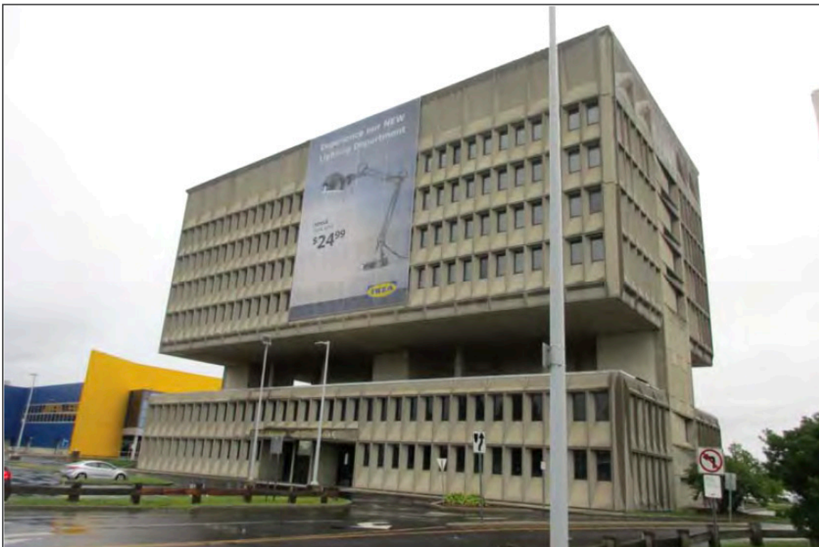
2. East and north elevations, facing southwest
