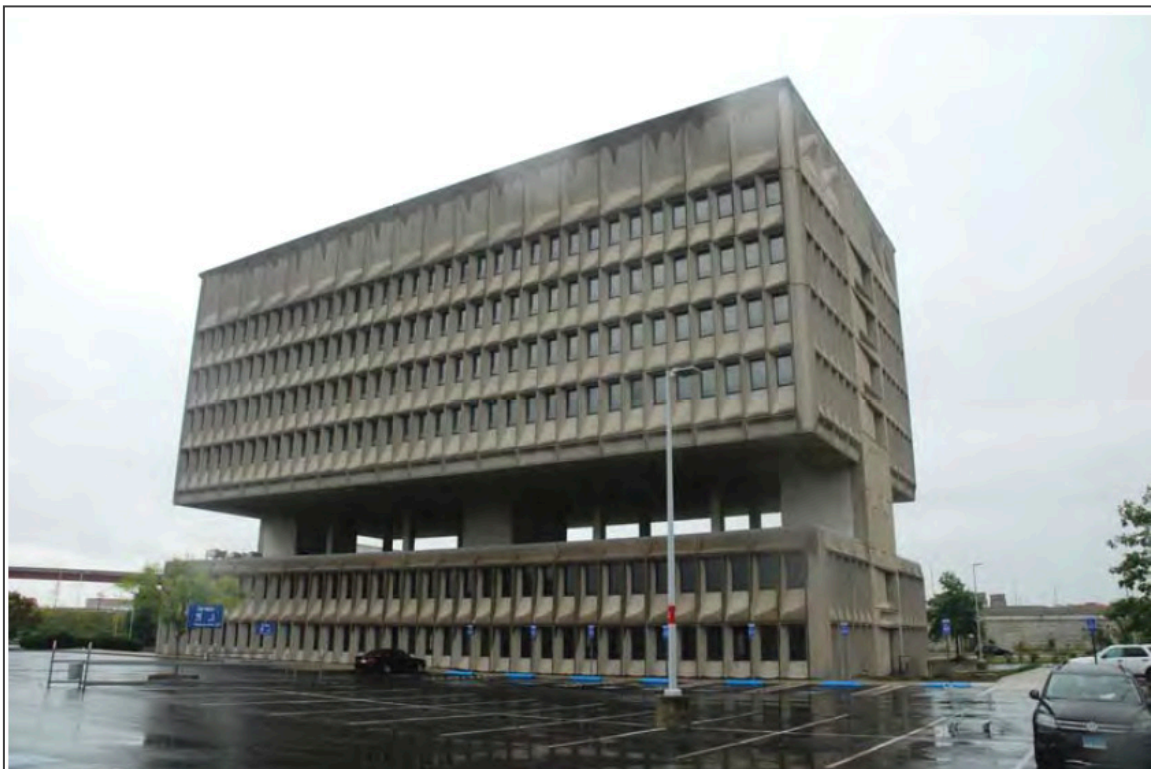
8. South and west elevations, facing northeast
