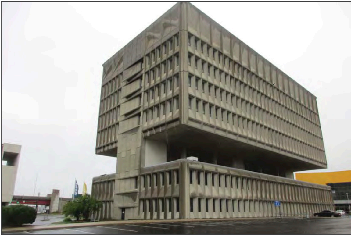
9. West and north elevations, facing southeast
