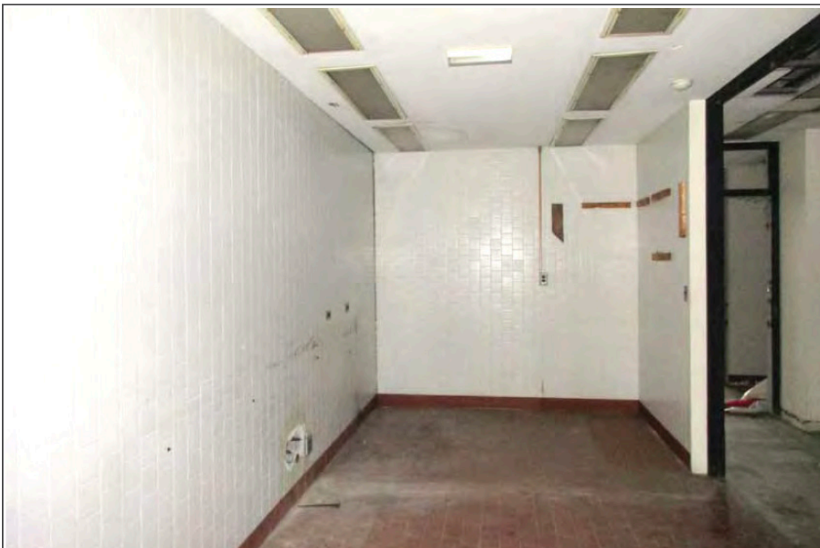
24. Eighth floor, former kitchen space
