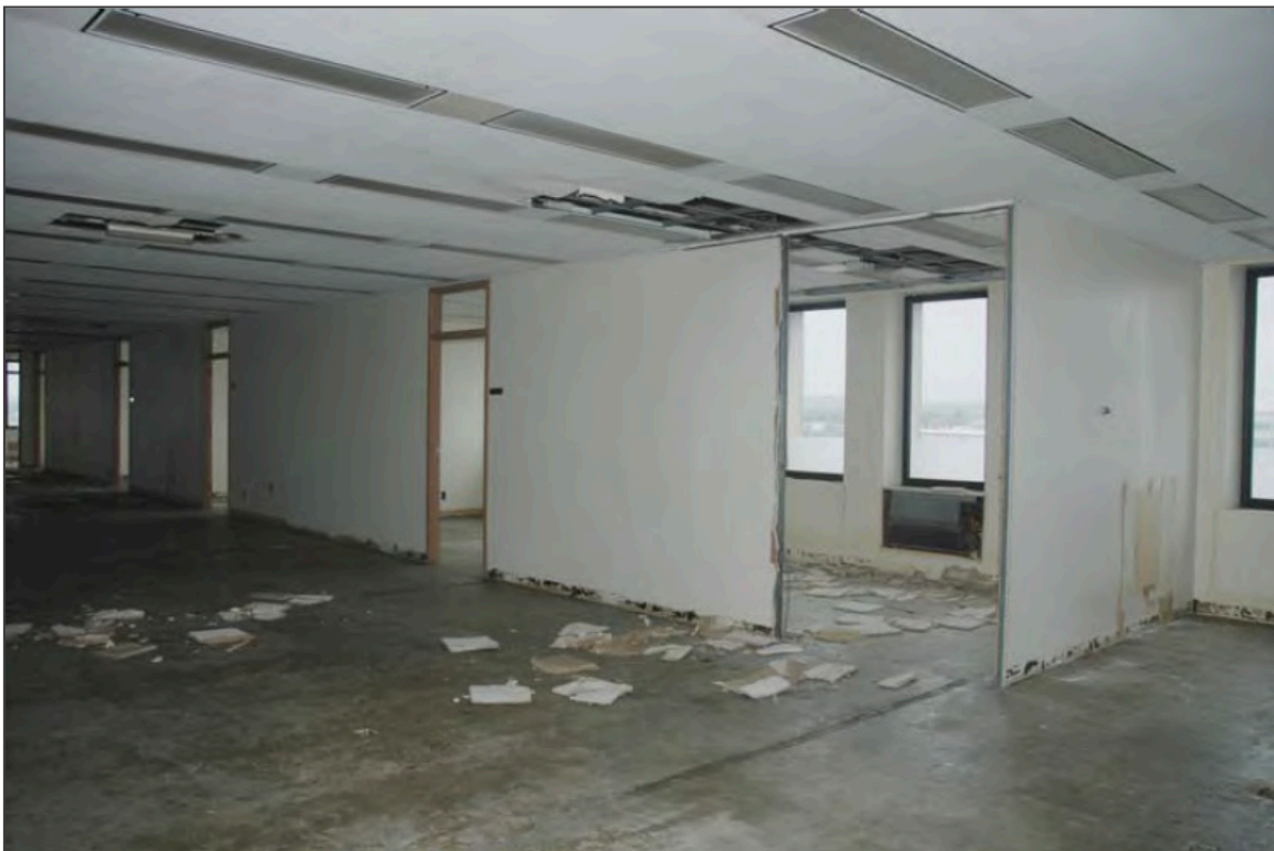
20. Seventh floor corridor, view towards former offices
