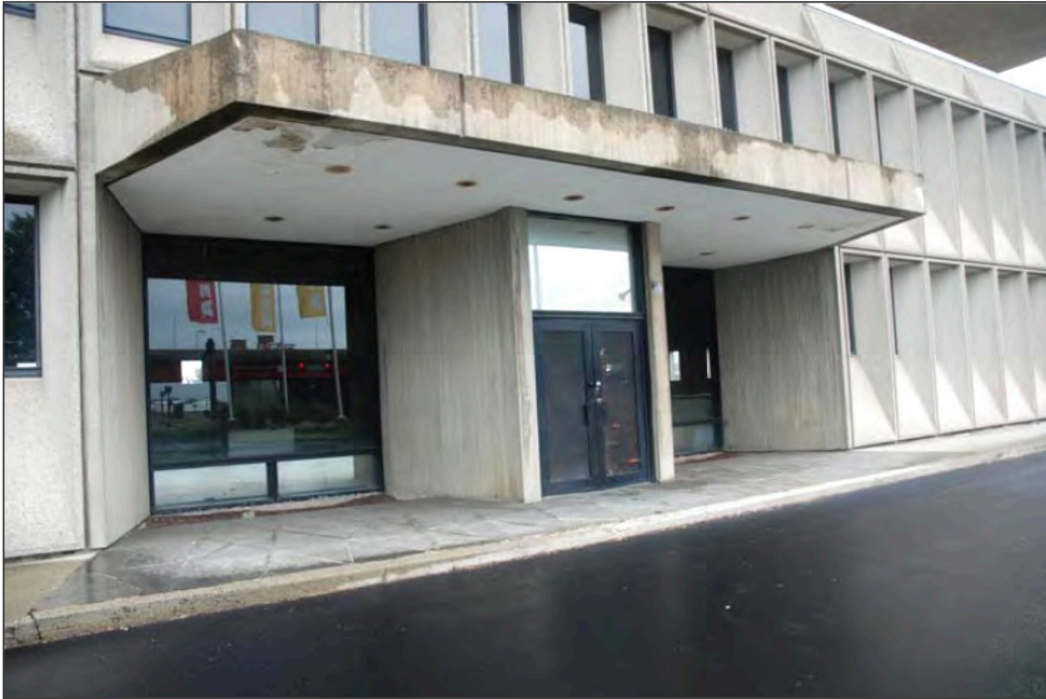
5. East elevation entrance, facing northwest
