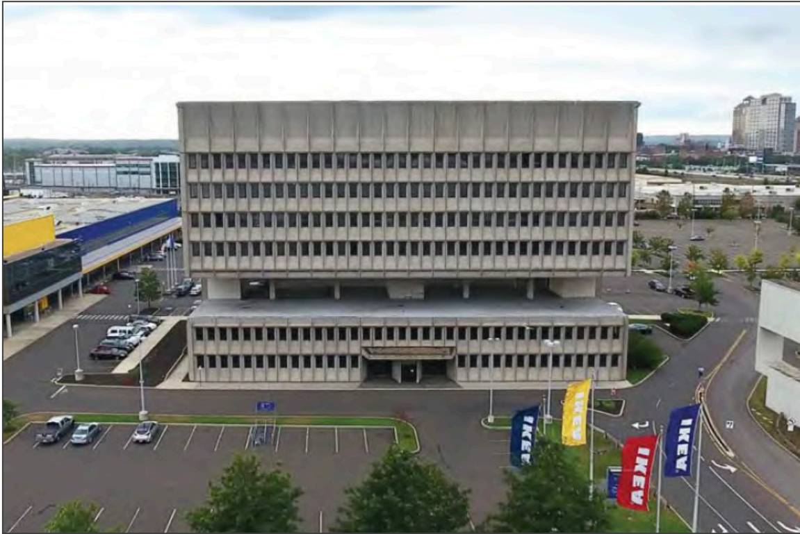
1. East elevation, facing west
