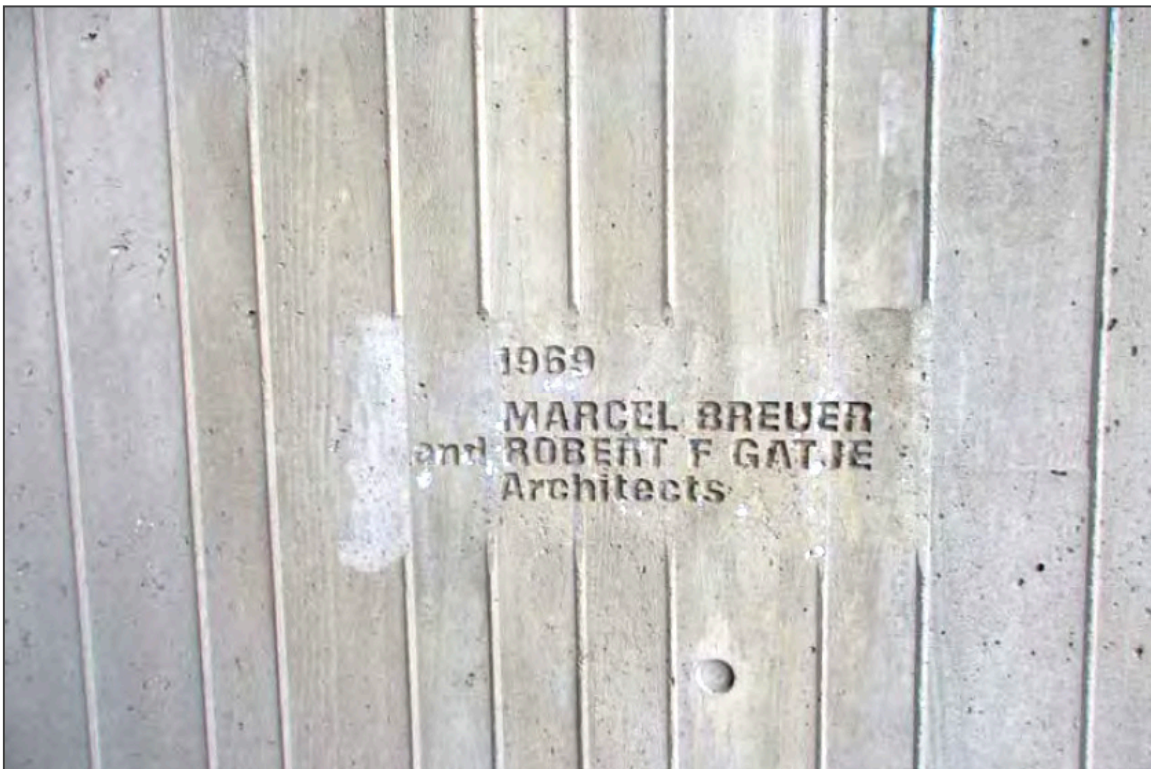
6. East elevation detail - date stamp and architect information
