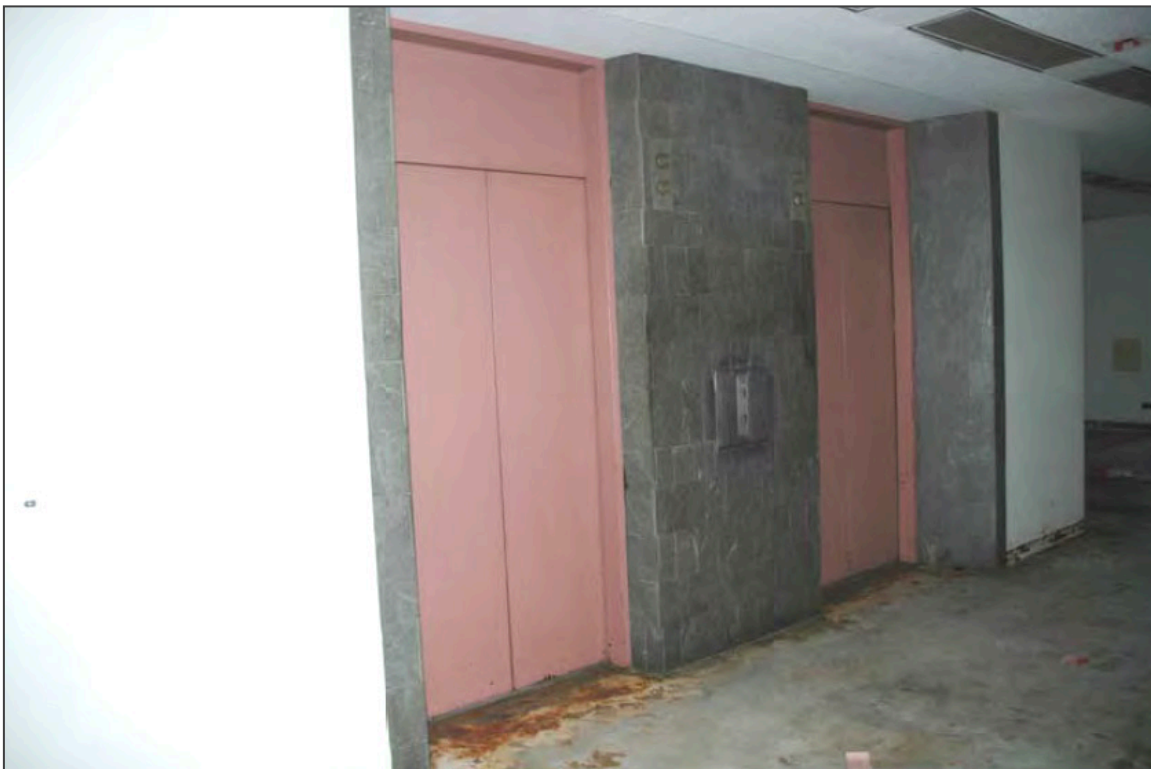
16. Sixth floor elevator lobby
