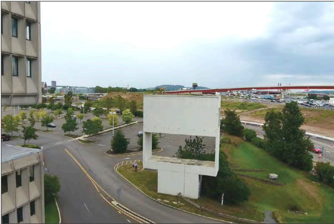
3. Sign structure south elevation, facing north
