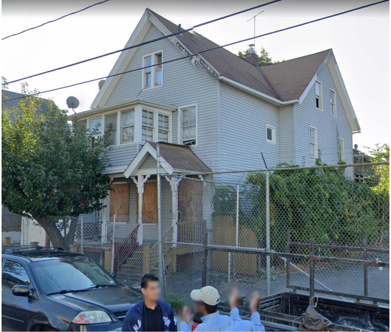
Streetview of 79 Garden Street, facing southwest (google, October 2019).
