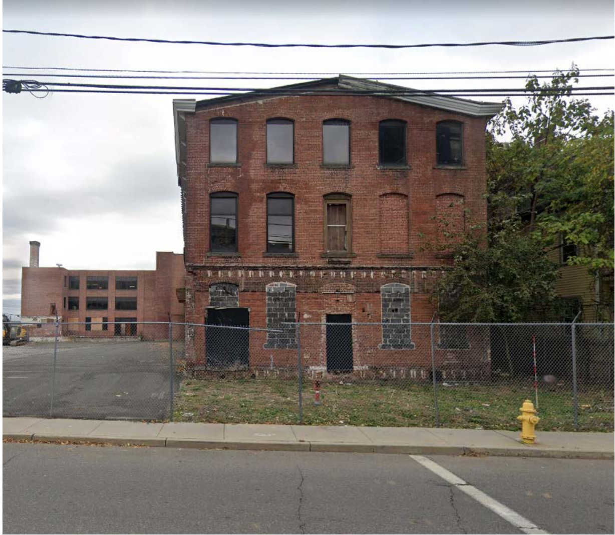
Streetview of 650 Atlantic Street, facing east (google November 2019).
