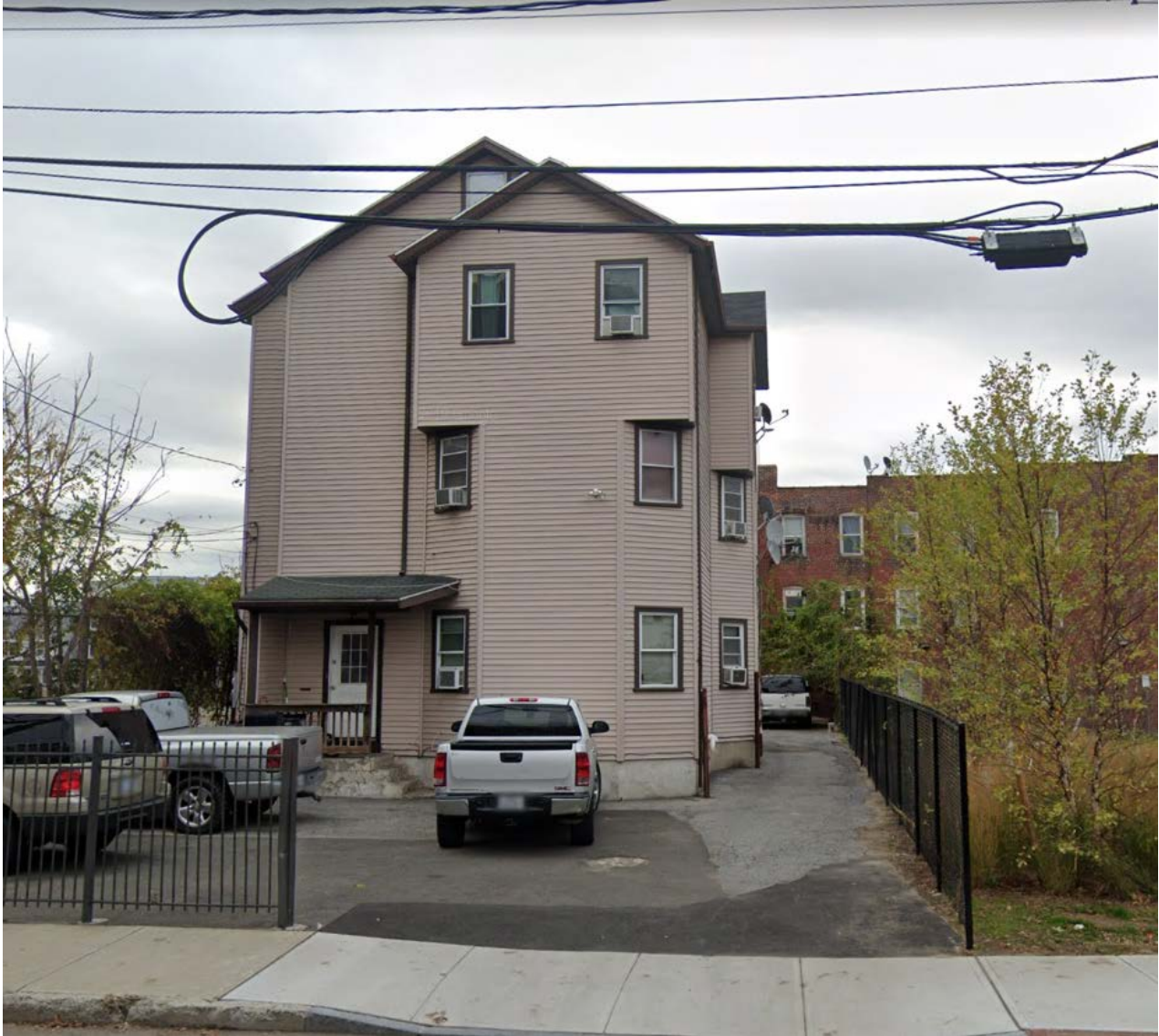
Streetview of 736 Atlantic Street, facing east (google, November 2019).
