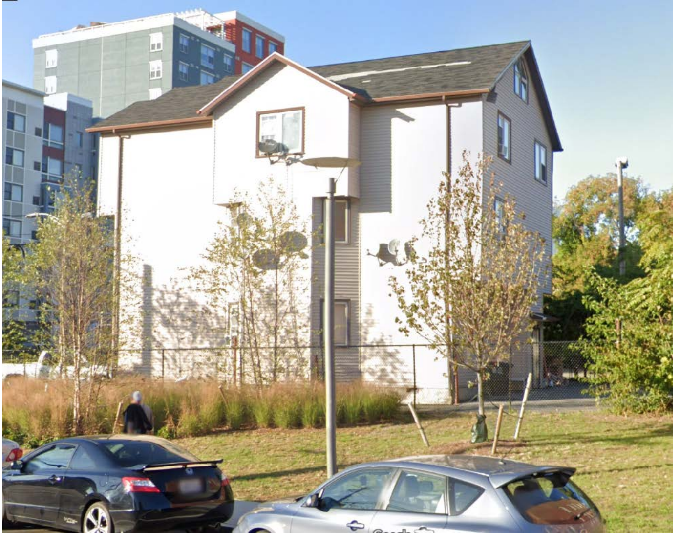
Streetview of 736 Atlantic Street, facing north (google, October 2019).
