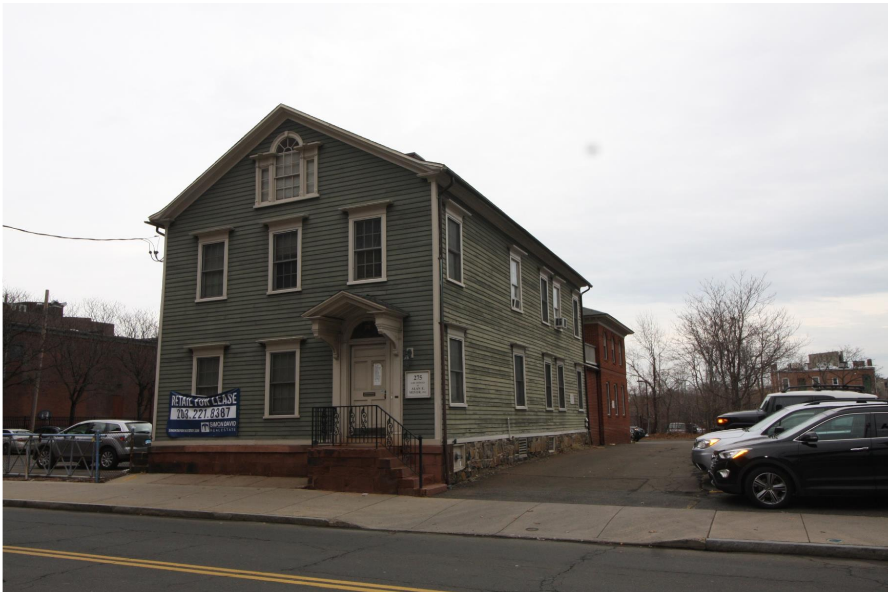
Photograph 1A. Front (western) and southern elevations as viewed from the west.
