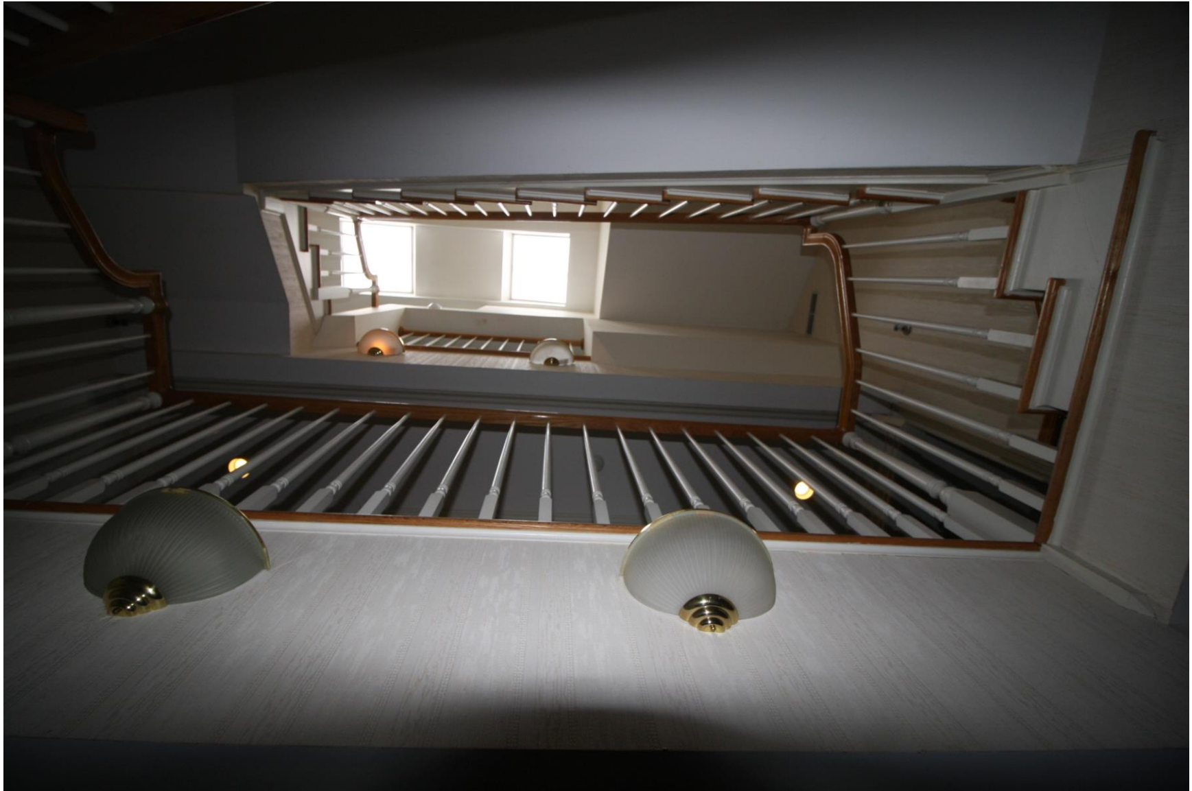
Photograph 10A. Modern replacement for the central stairwell on southern side of building. (Room 5 on HABS/NRHP nomination plan.)
