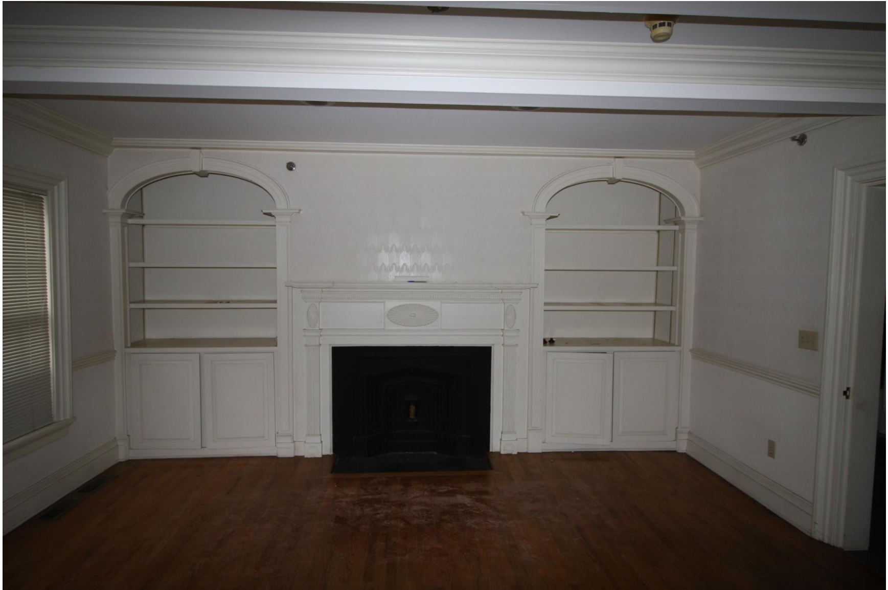
Photograph 6A. Interior elevation of north wall, first-story front room
