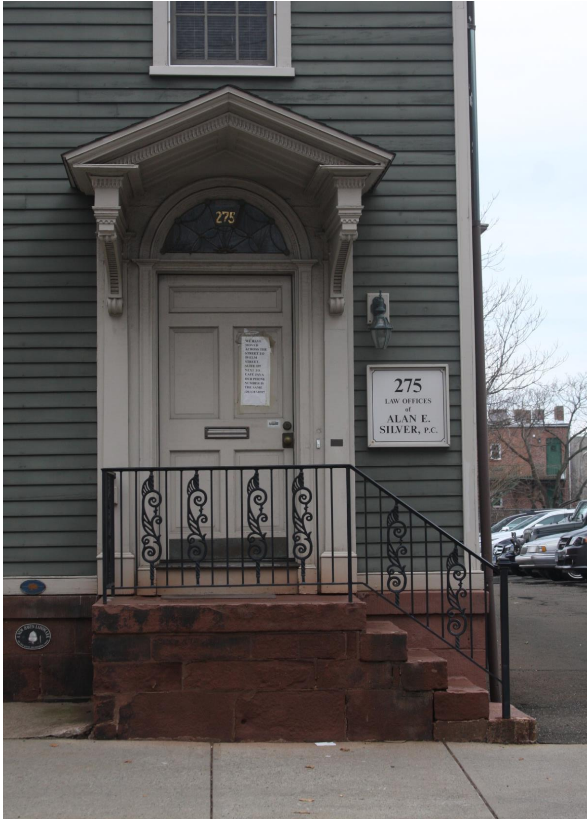
Photograph 3A. Front entry as viewed from the west.
