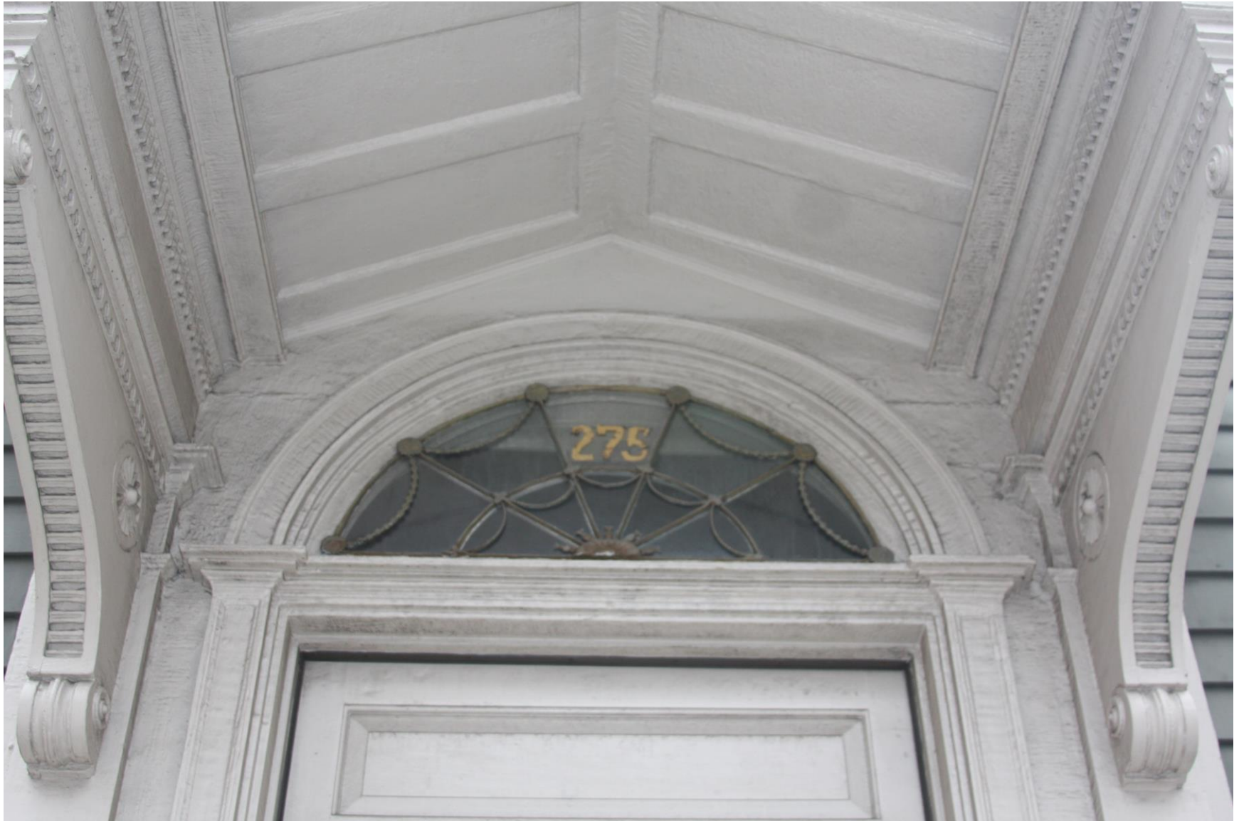
Photograph 4A. Close-up view of front entry fanlight transom.
