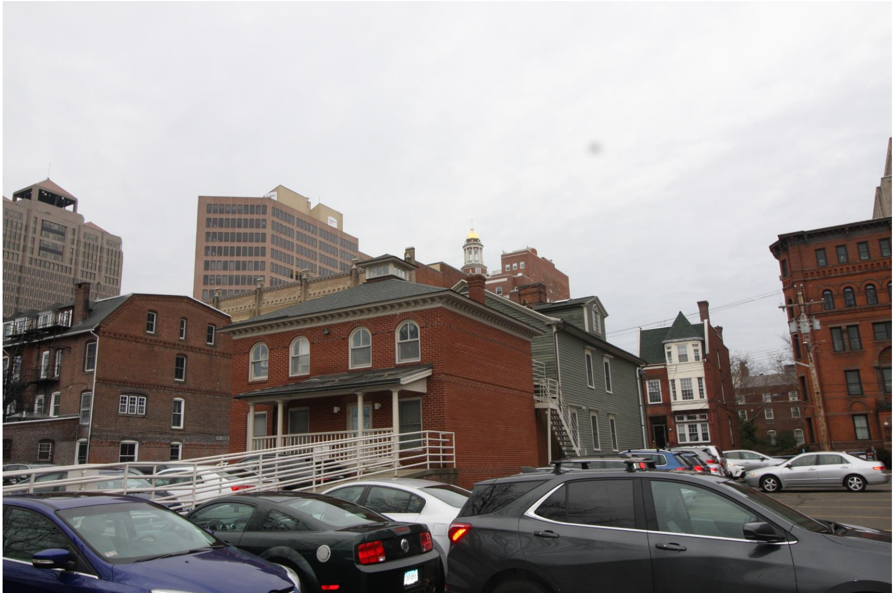
Photograph 2A. Rear (eastern) and northern elevations as viewed from the northeast.
