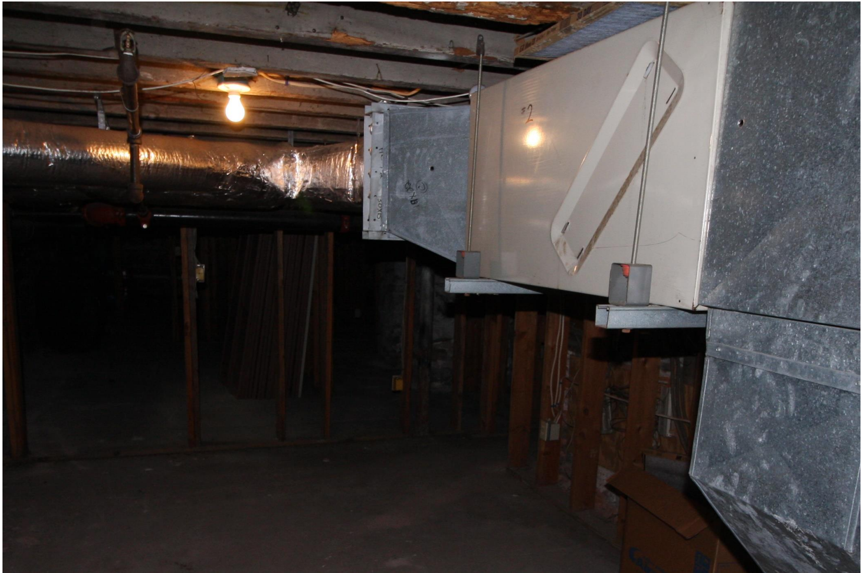
Photograph 18A. Looking towards the chimney NRHP nomination.
