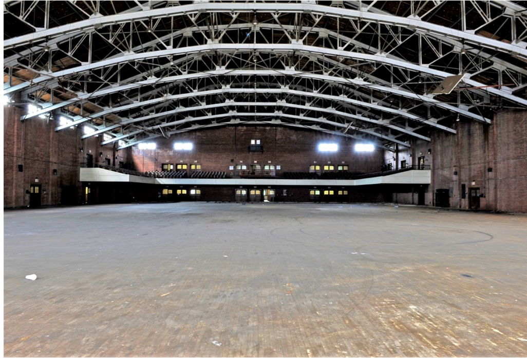
44. Drill Hall Interior looking North to spectator's gallery/ balcony, circa 2009.
