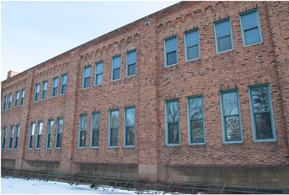
8. West elevation, facing Northwest.
