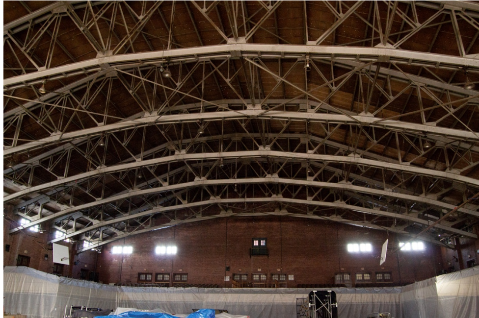
42. Drill Hall Ceiling wide view detail looking towards spectator balcony.
