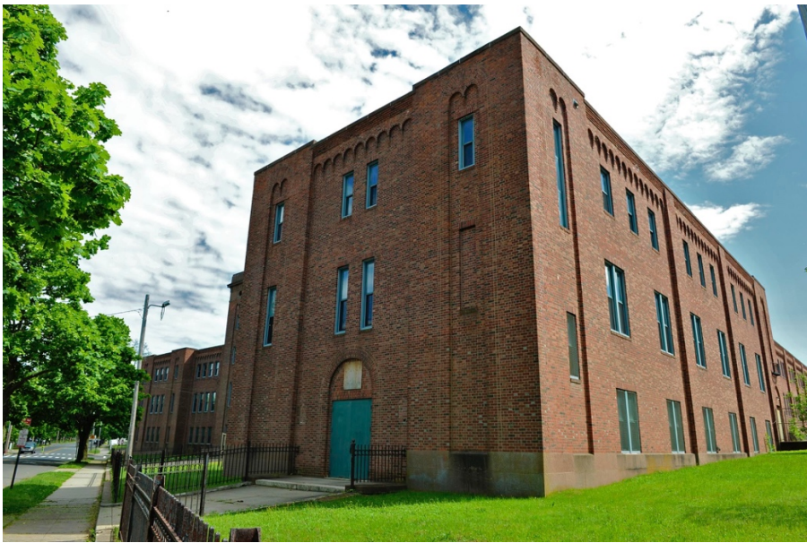
7. Foot Guard Wing West Façade / Tower, Facing Southeast.
