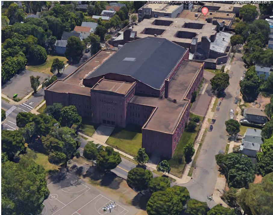
Figure 5. Facade, Facing South ( Google Earth , September 2019).
