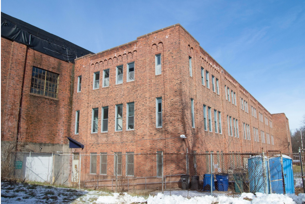
12. Rear of East elevation.
