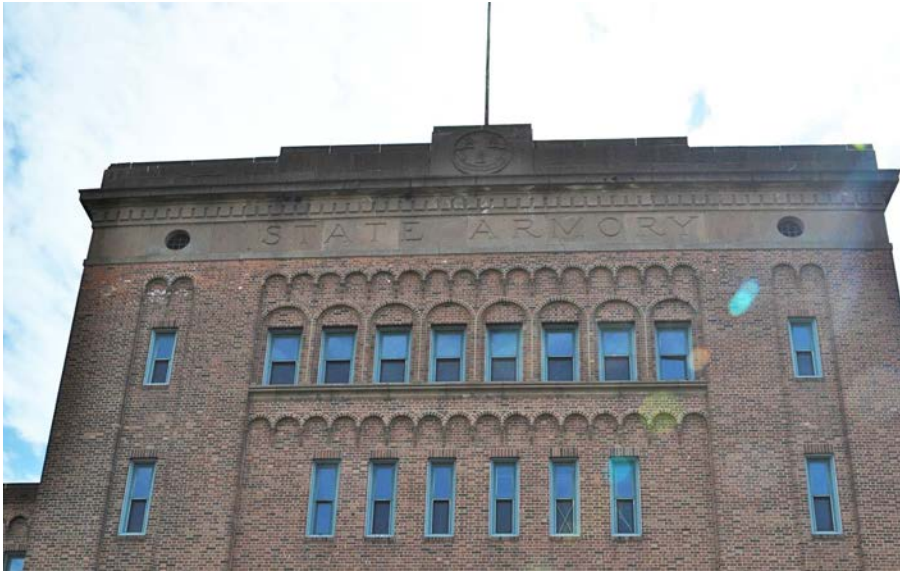
4. Entry Tower, facing South..
