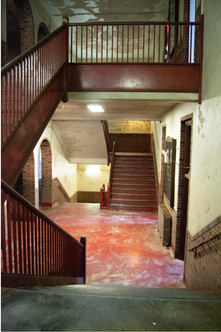
20. Main stairwell descending view to second floor landing.
