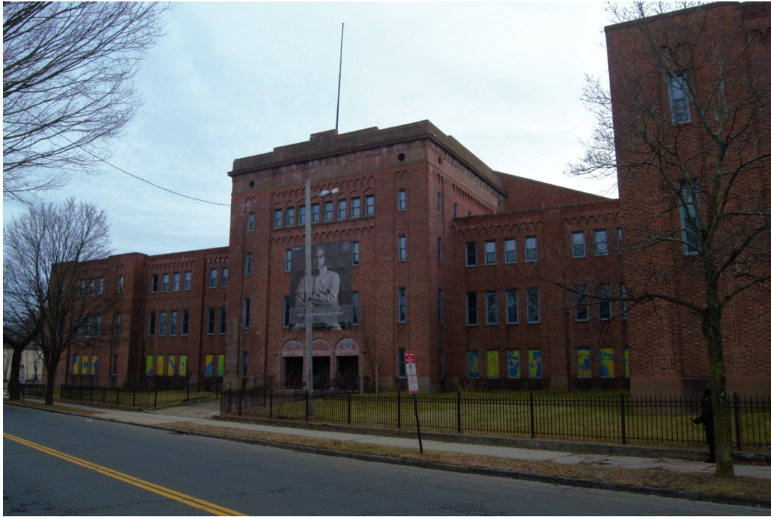
1. Façade, North Elevation, facing South.
