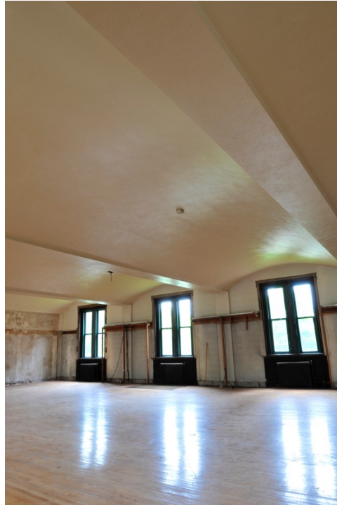
38. Foot Guard Ballroom ceiling detail, circa 2009.
