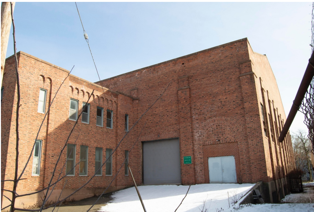
13. Rear of West elevation with garage entry to Drill Hall.
