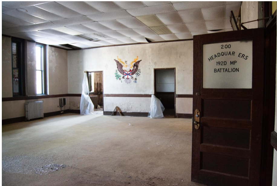
29. Central Headhouse, Officer's Club, Second Floor Bar area.
