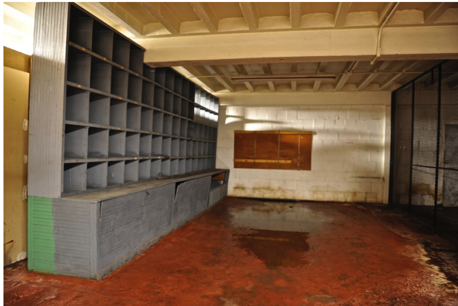
39. Supply Room, Ground Floor, circa 2009.
