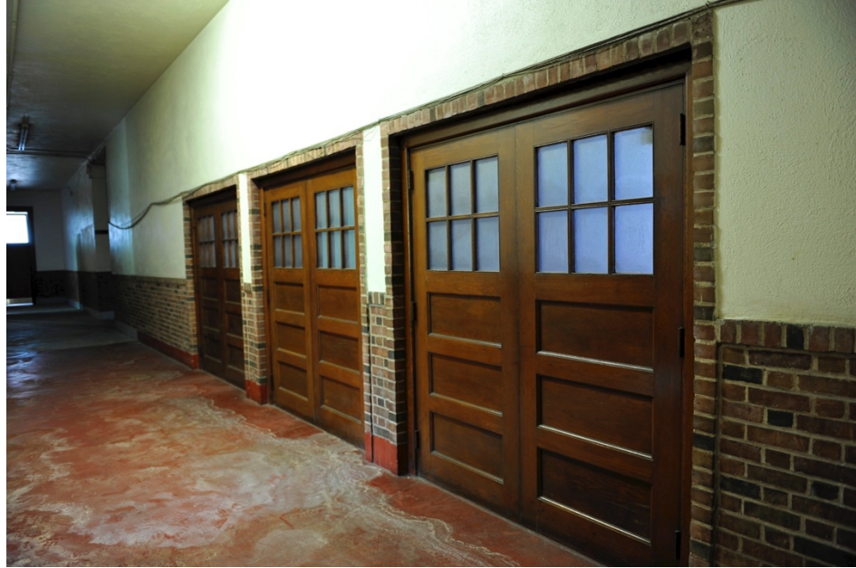
32. Set of double wood Doors leading to Drill Hall, circa 2009.
