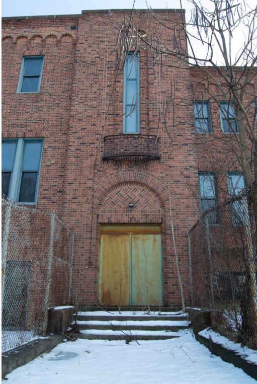
6. West Elevation Tower, Foote Guard Wing, Balcony.
