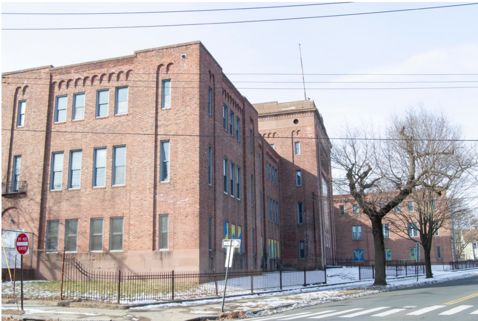
9. East elevation looking West, East Tower.
