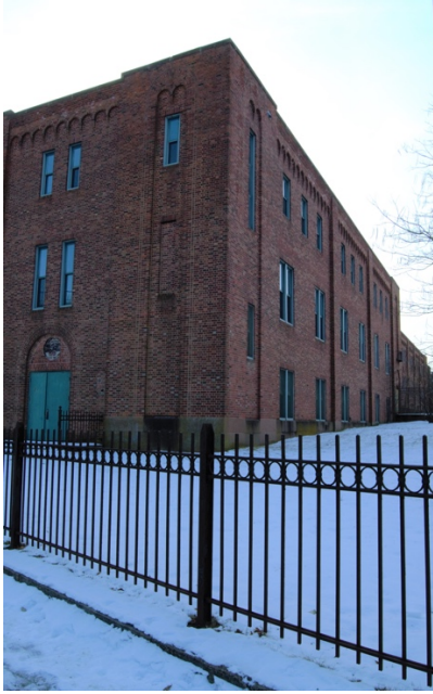
10. Foot Guard Tower facade and West elevation, facing Southeast.
