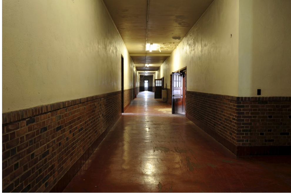
46. Hallway/ Corridor Detail, Second Floor, circa 2009.
