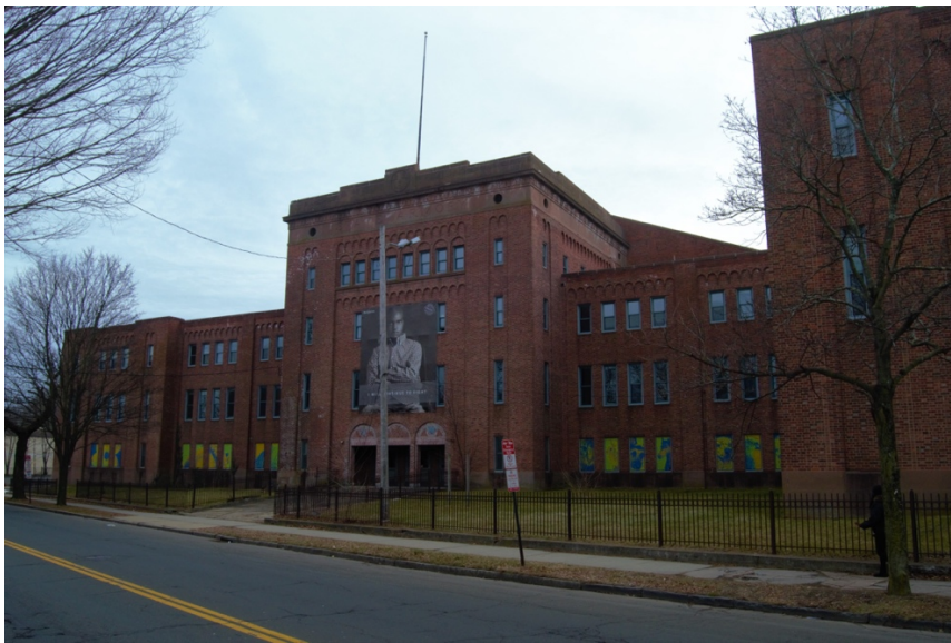
2. Façade, facing Southeast down Goffe Street.
