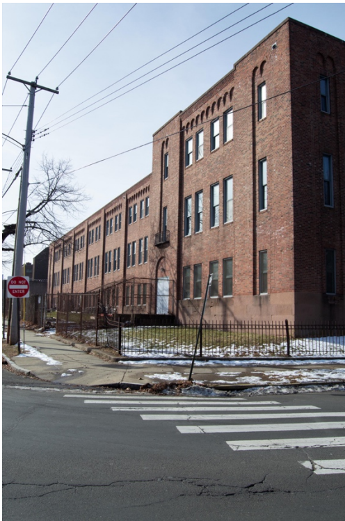
11. East Tower, facing Southwest.
