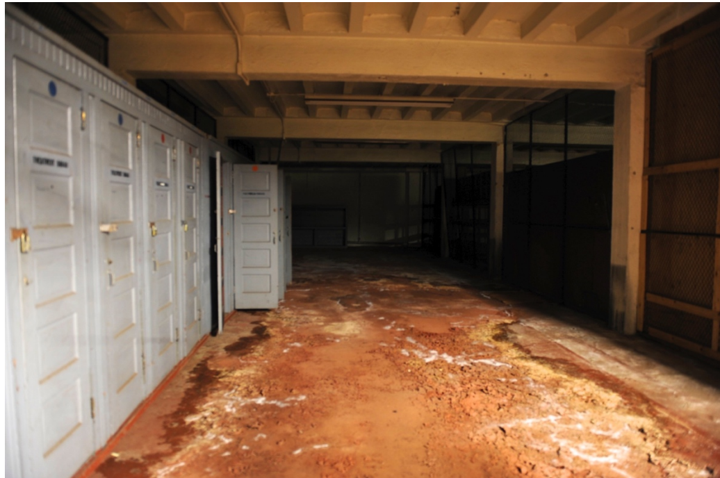
41. Unit storage area, Ground floor, circa 2009.
