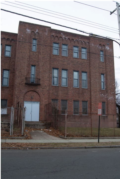
5. East Corner Tower, East Elevation, Facing West.
