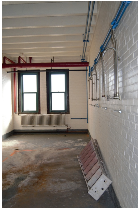
27. East Wing, Ground Floor, Showers (part of latrine area).
