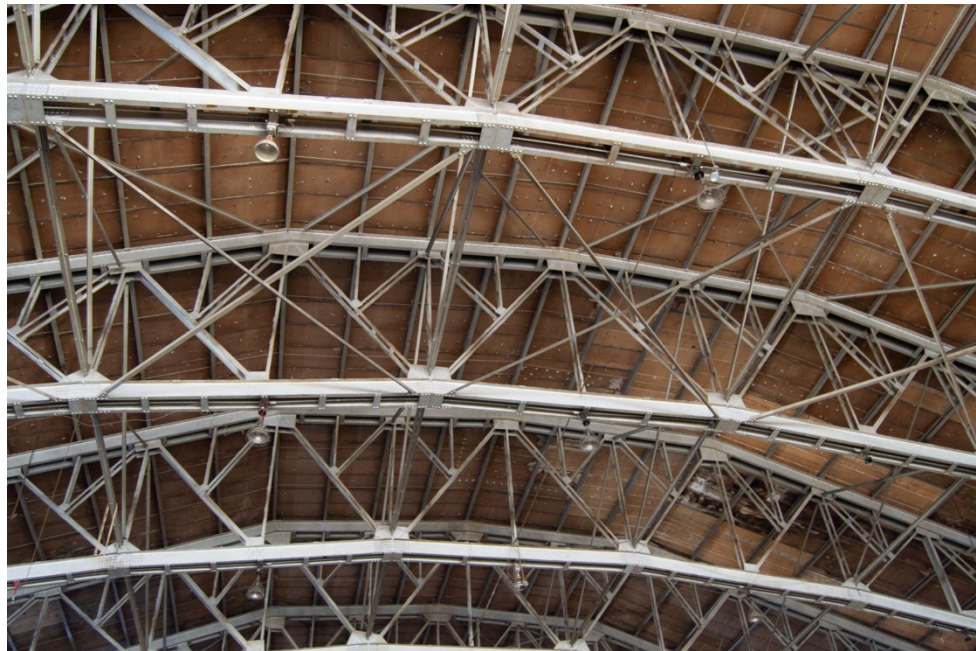
43. Drill Hall Ceiling detail.
