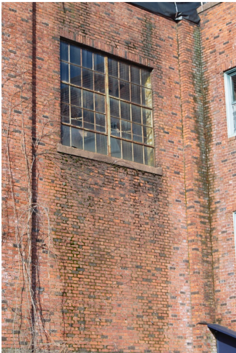
15. Rear casement windows, facing Southwest from County Street.
