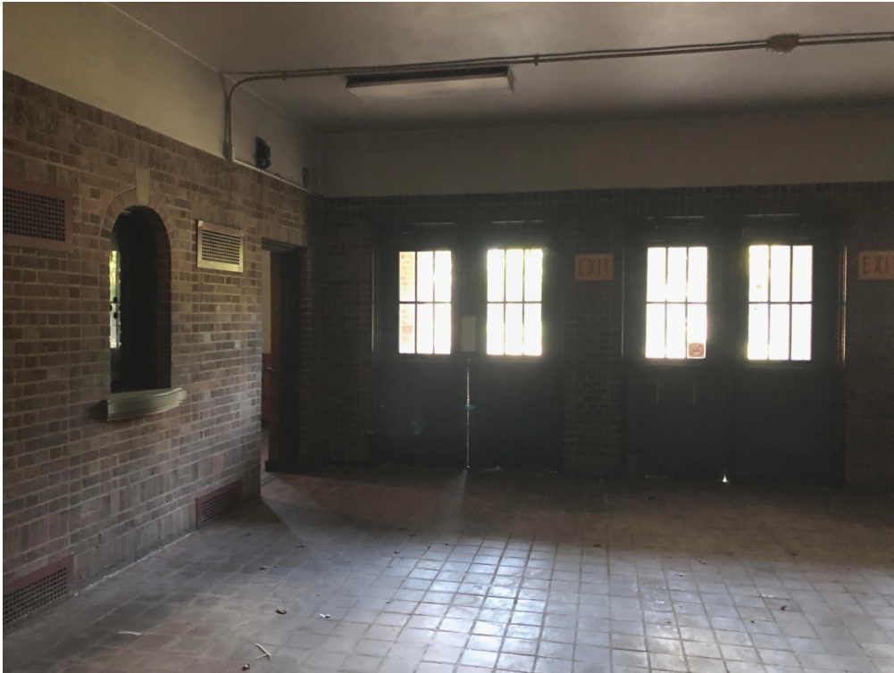
19. Foyer, Ground Floor.
