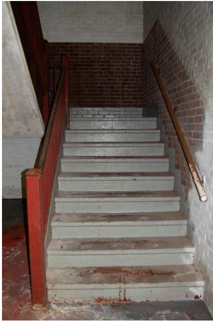
22. Secondary Stairwell, east side of Headhouse.
