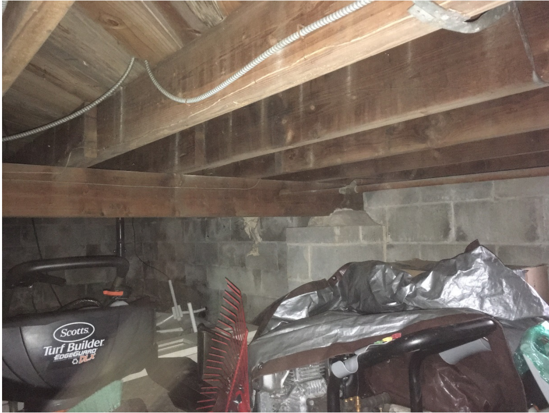
Detail of crawl space, 12/2/20.
