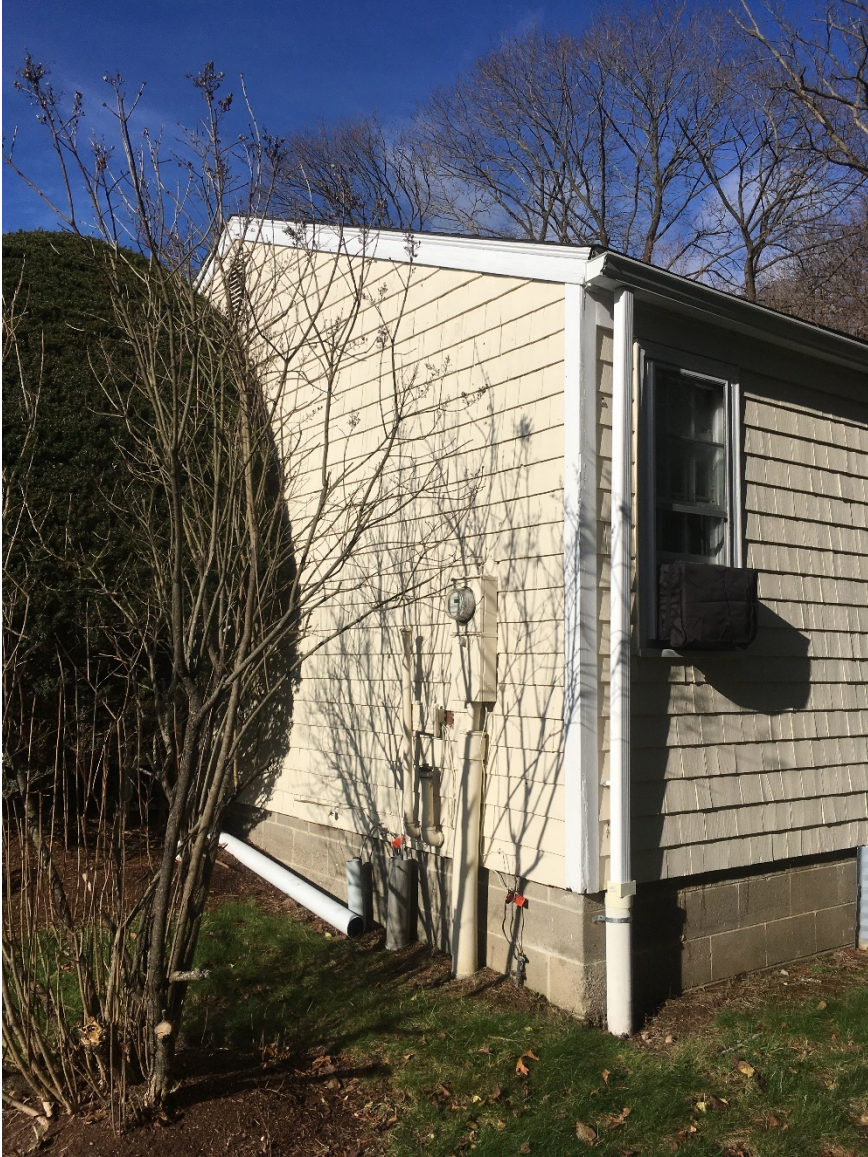
Detail of concrete block foundation and south (side) elevation, 12/2/20.
