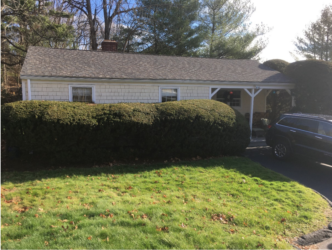
Façade (west elevation), view looking east, 12/2/20.
