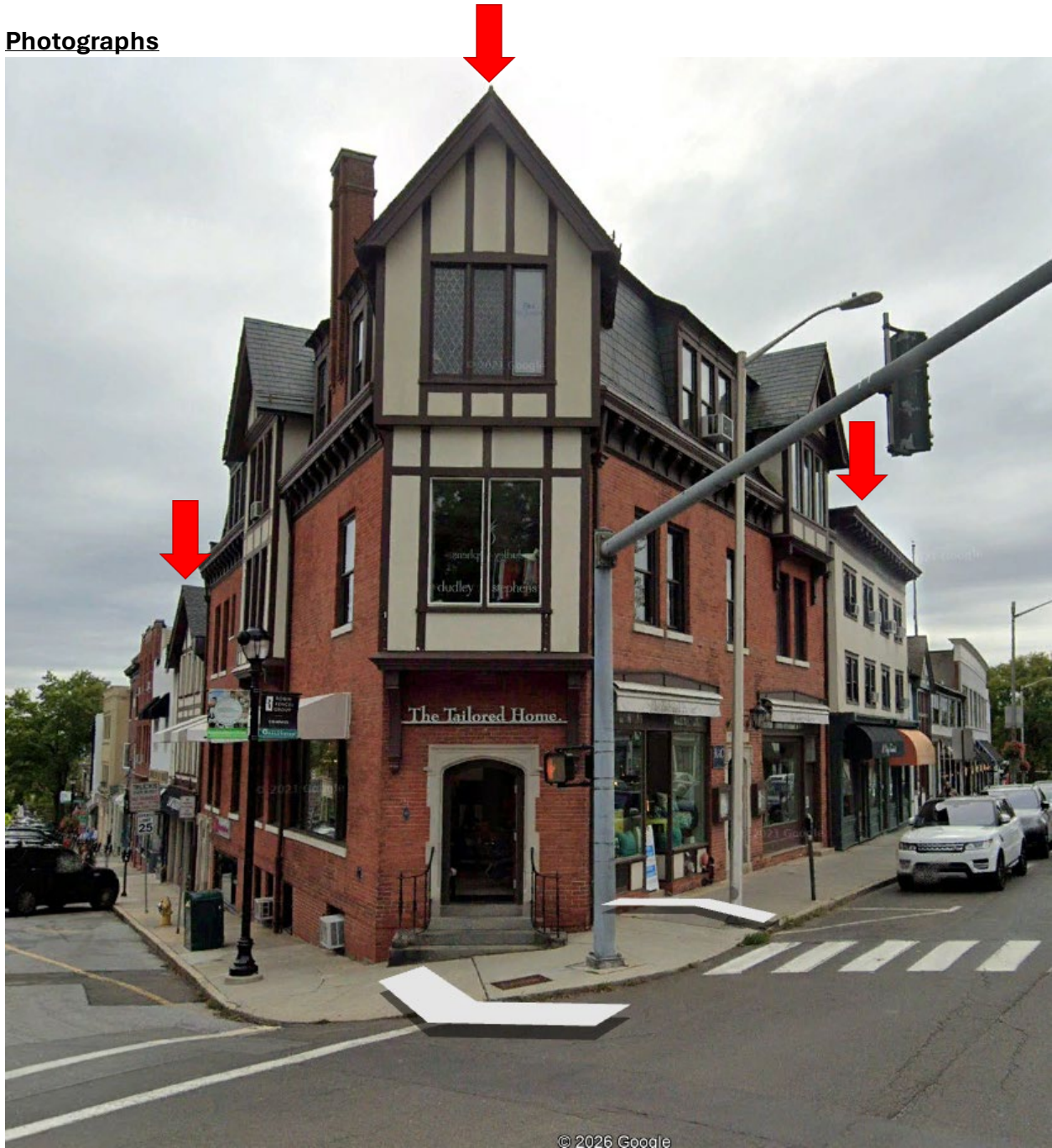
2 Greenwich Avenue (center), 10 Greenwich Avenue (left), and 10-12 West Putnam Avenue (right), Greenwich, view looking south. Google Earth , October 2019.
