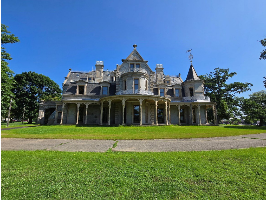
Photograph 1. Lockwood Mathews Mansion, exterior, view north.
