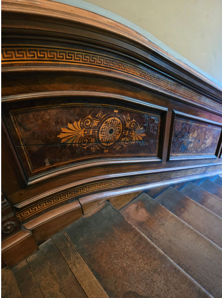
Photograph 38. Grand Staircase detail, view northwest.
