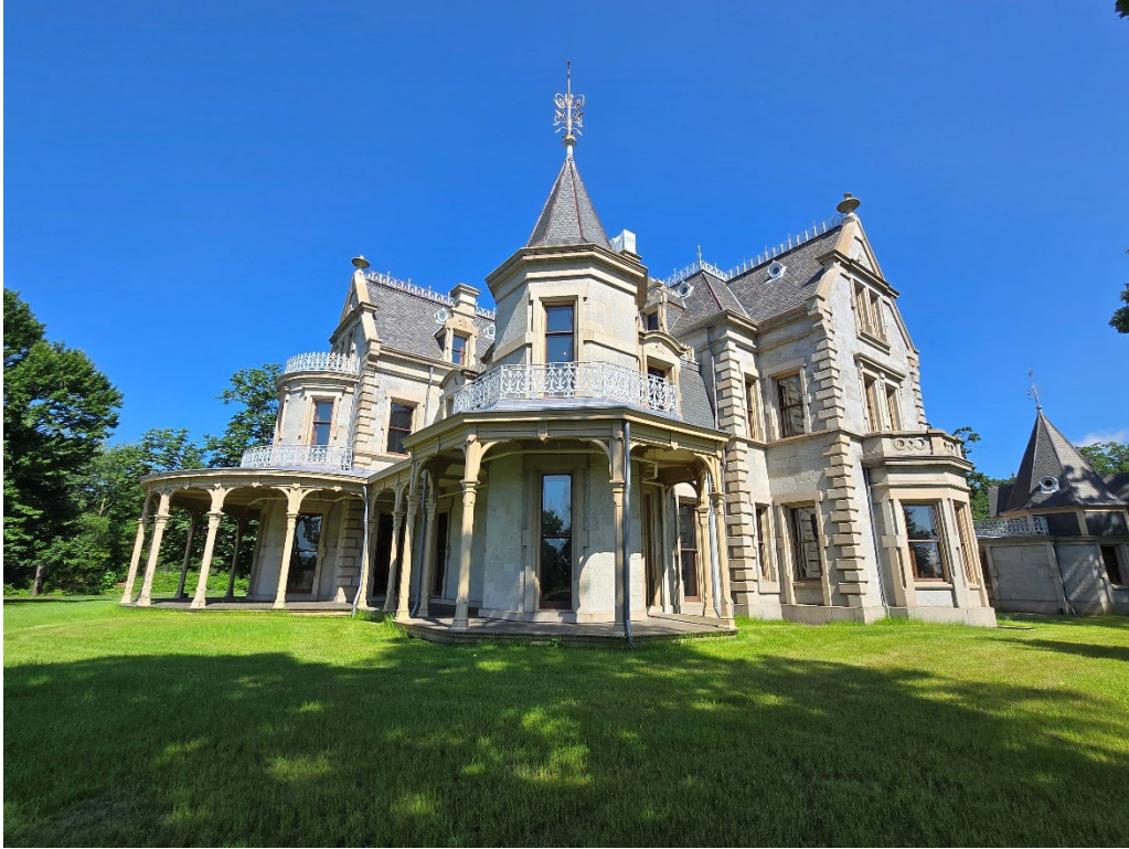
Photograph 5. Exterior, view northwest.
