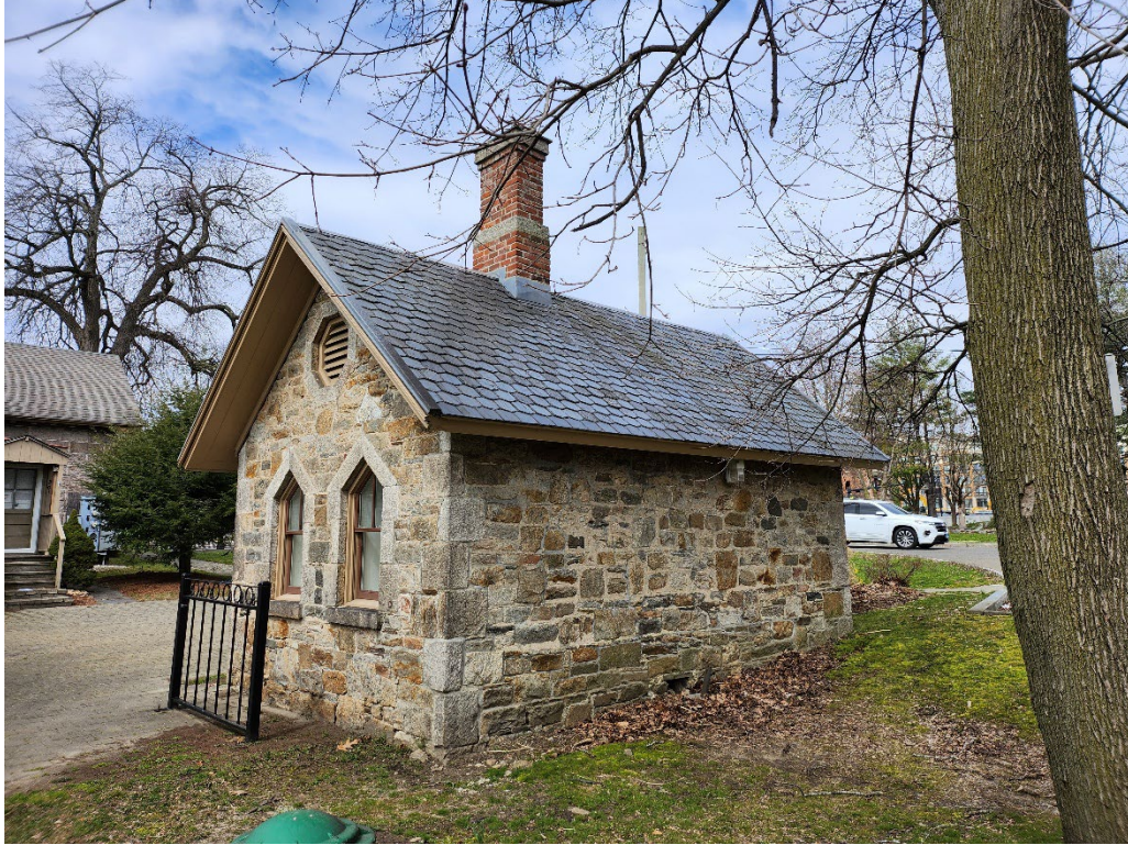
Photograph 84. Summer Kitchen, view west.
