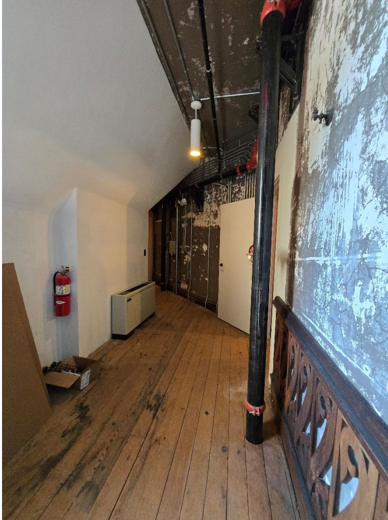
Photograph 56. Top of Servants' Stairs leading to third floor, view south.
