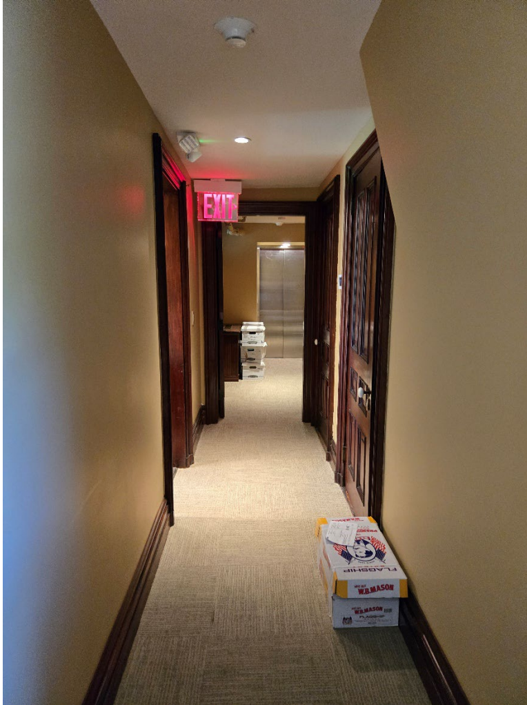
Photograph 42. Hallway on second story of Servant's Quarters, view south.
