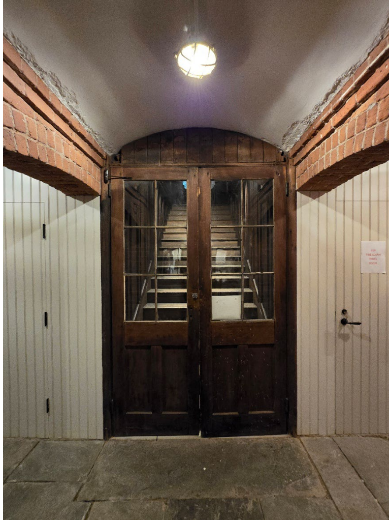
Photograph 66. Stairs leading to the Entrance Hall/Rotunda, view north.
