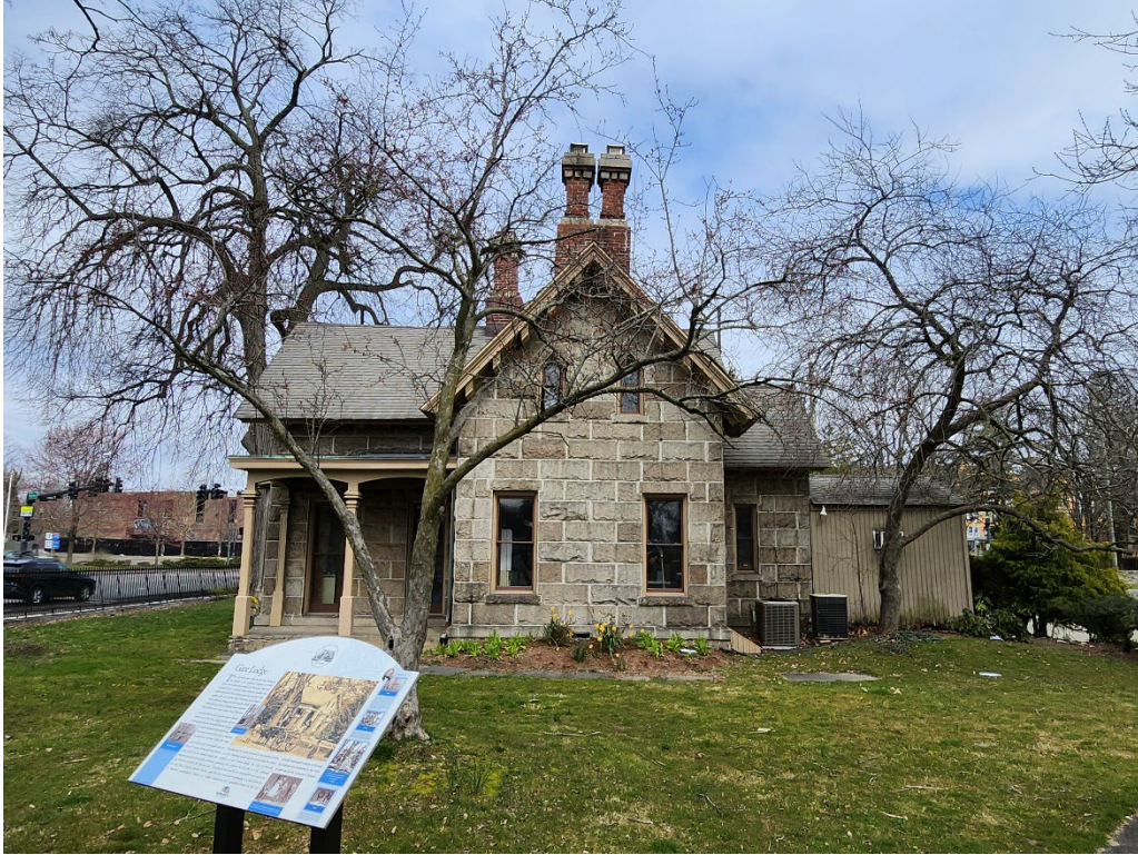
Photograph 71. Gate Lodge, southern elevation, view north.
