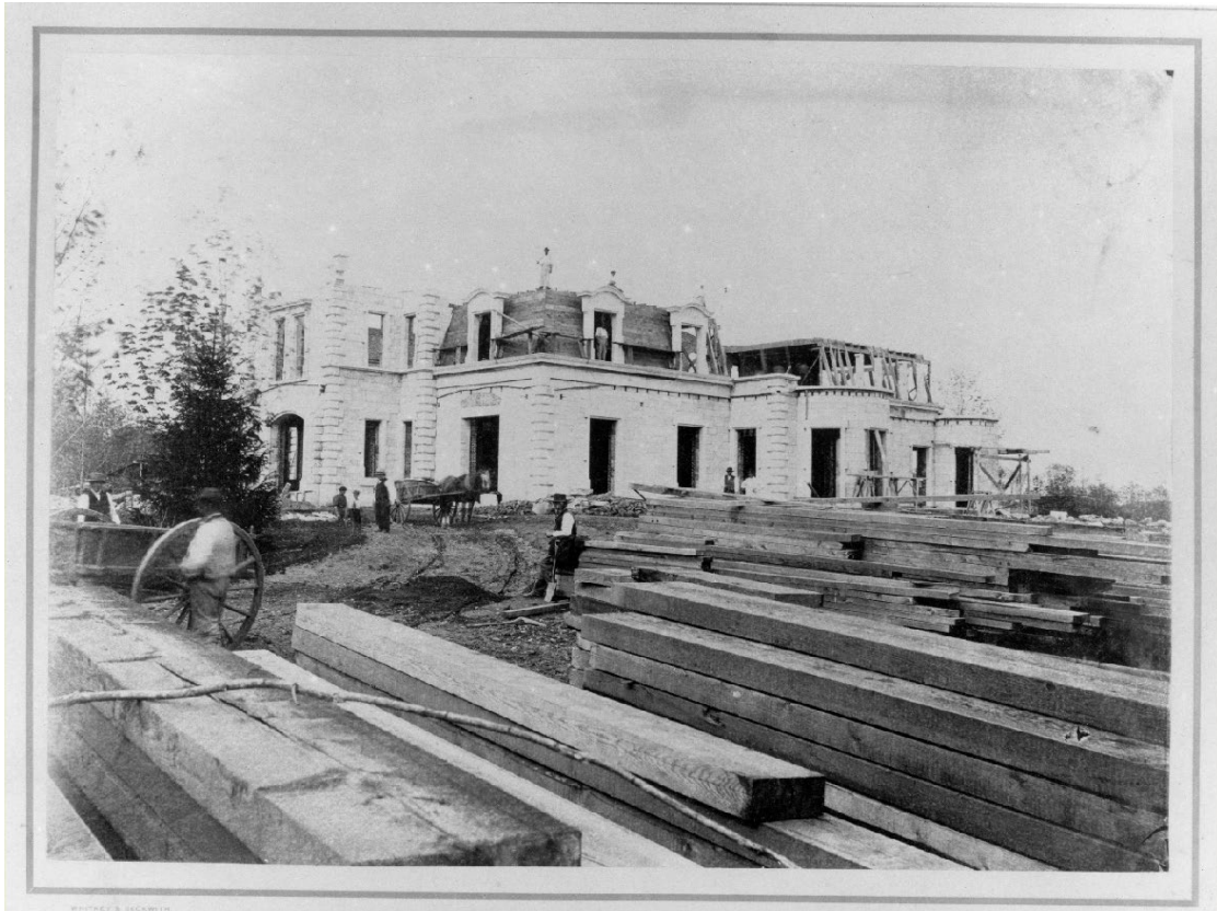
Figure 23. Construction of the mansion, c. 1865-1866 ( Lockwood Mathews Mansion Archives ).
