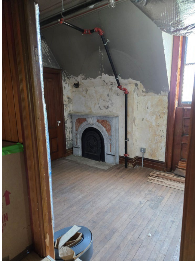
Photograph 59. Fireplace in third floor bedroom, view southeast.
