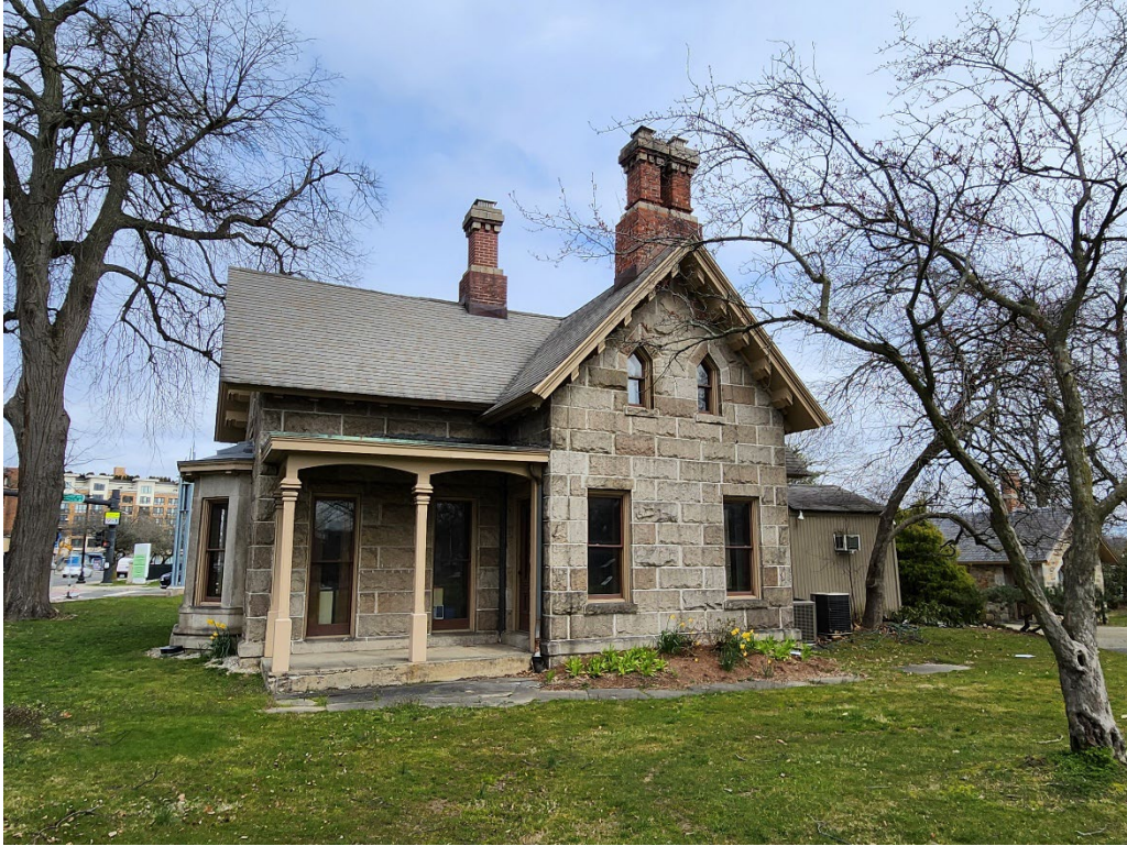
Photograph 73. Gate Lodge, northern elevation, view south.
