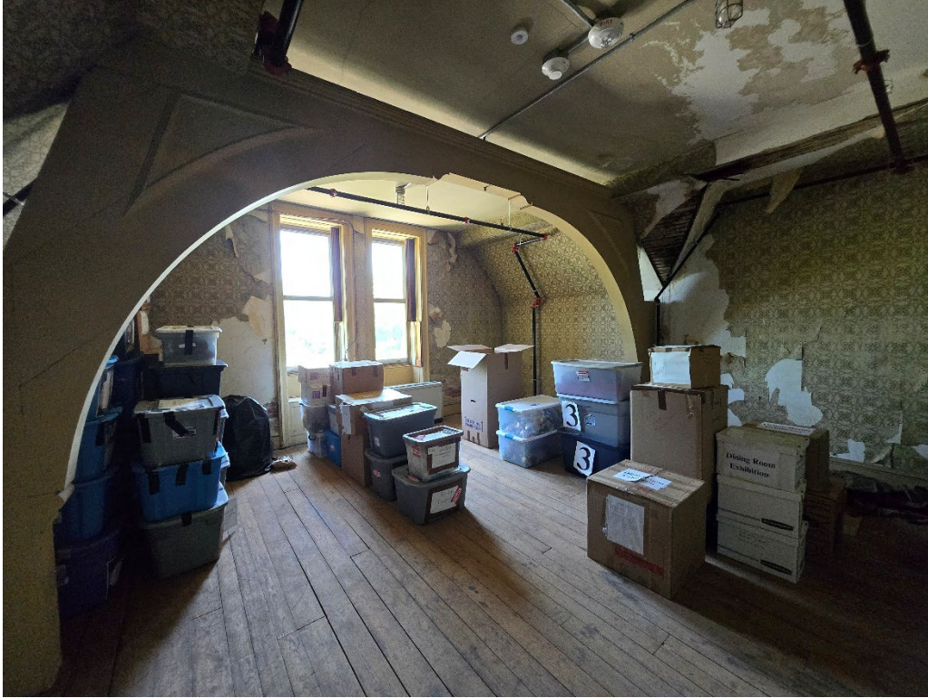
Photograph 57. Room on third floor, view northeast.
