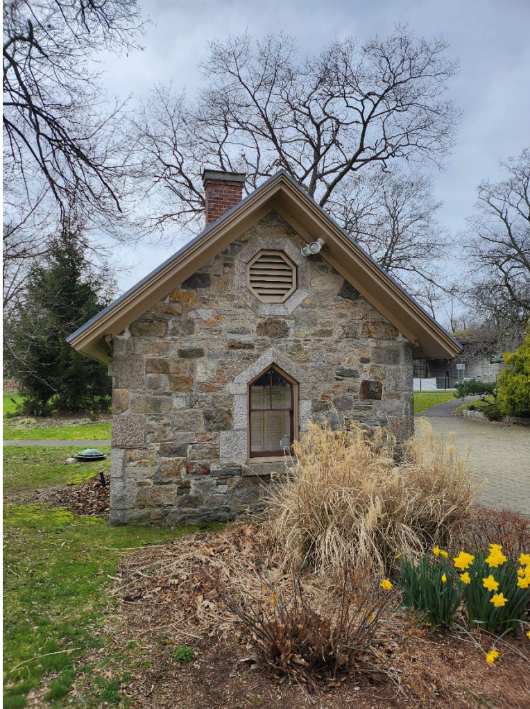
Photograph 81. Summer Kitchen, view south.
