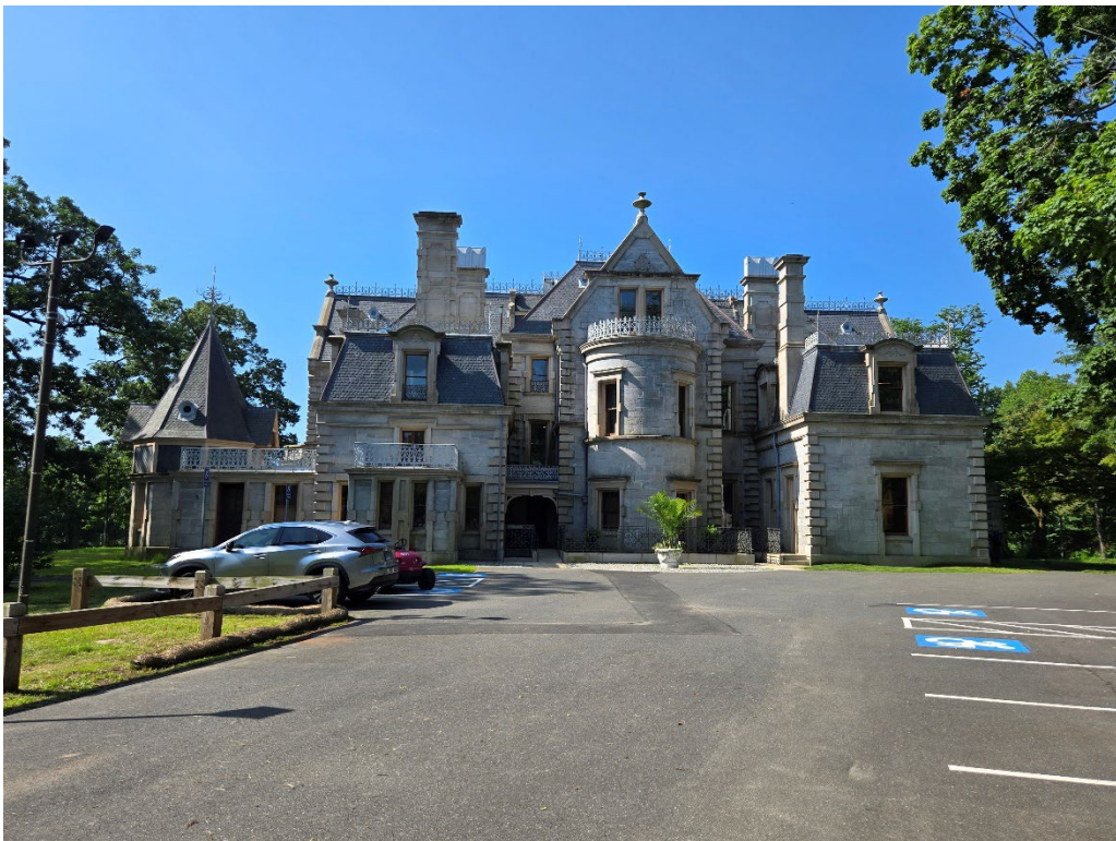
Photograph 6. Northern elevation, view south.
