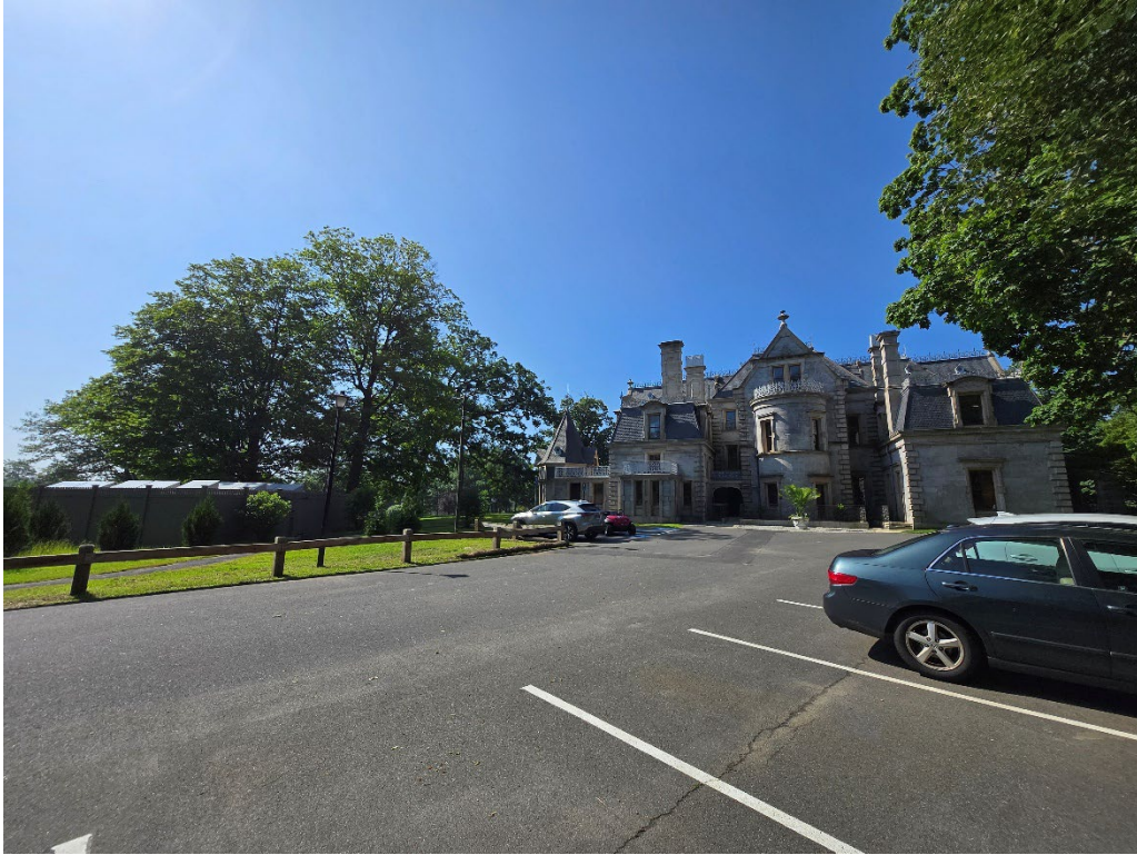
Photograph 94. Mechanicals in new housing, view southeast.
