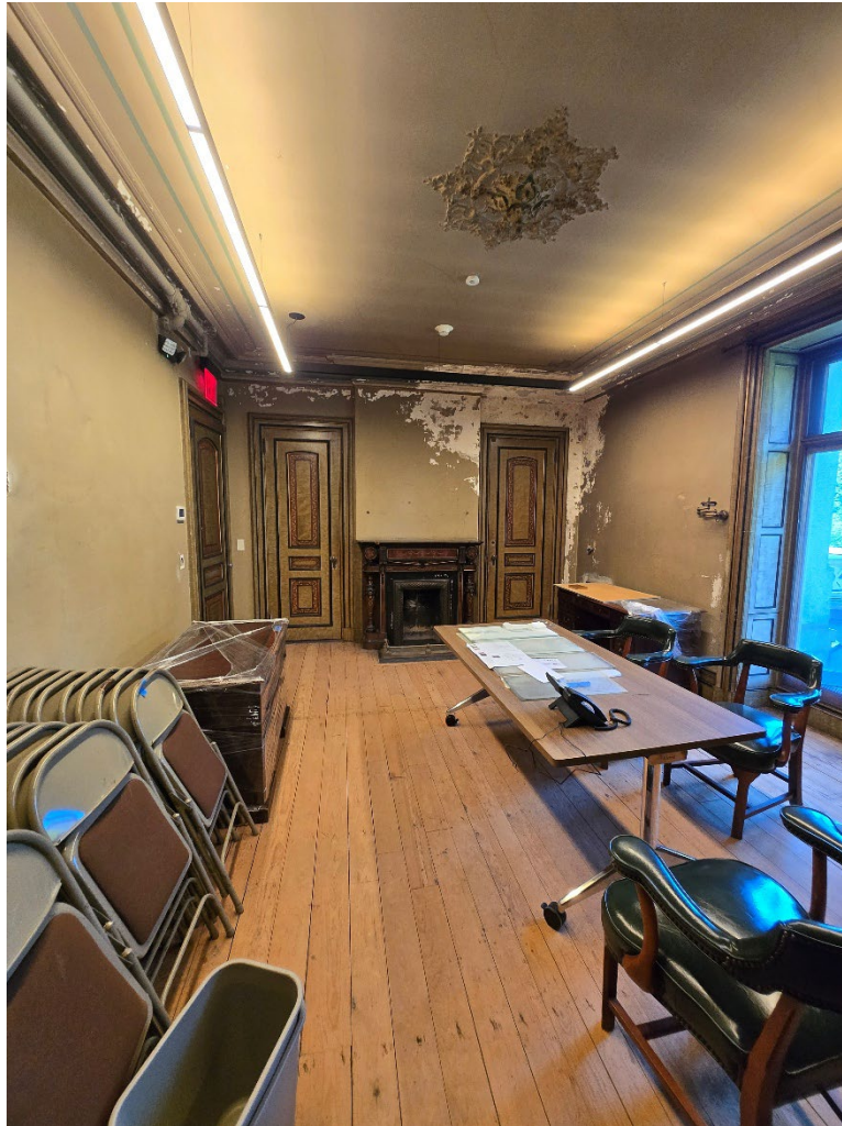
Photograph 54. Italian Suite, view south.
