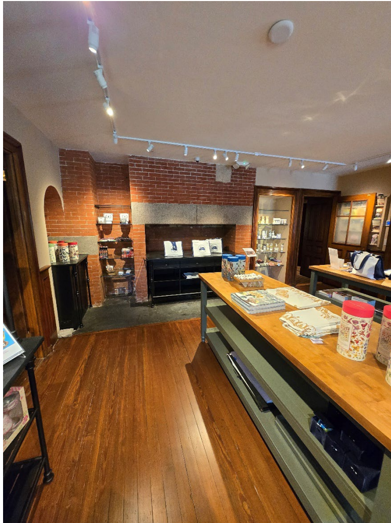
Photograph 18. Former kitchen area, view southeast.
