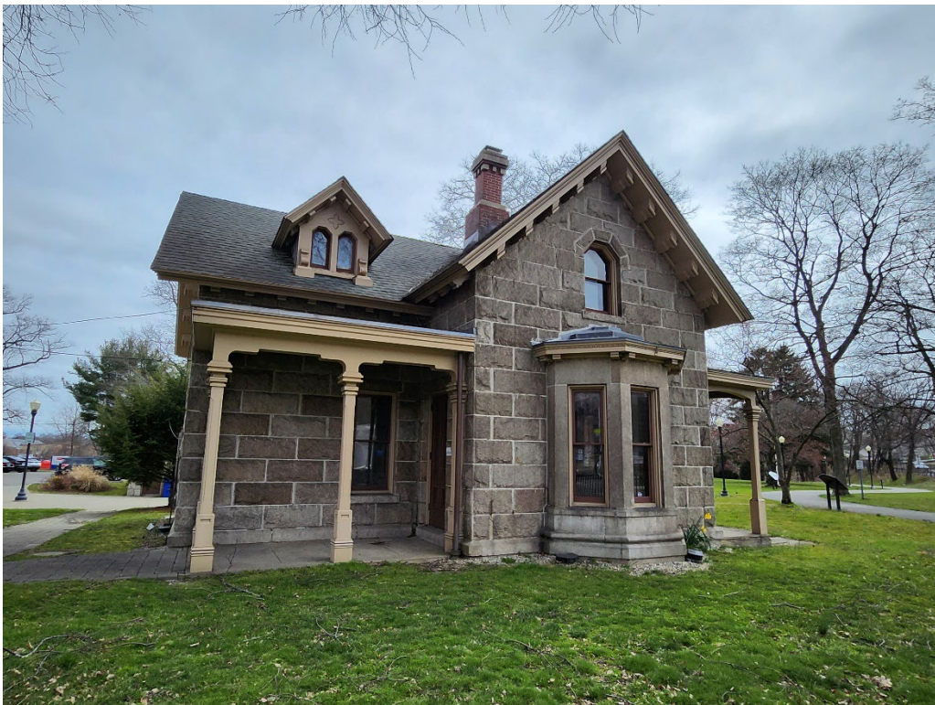
Photograph 72. Gate Lodge, western elevation, view east.
