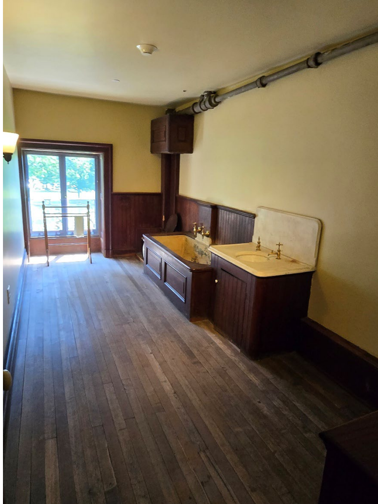
Photograph 36. Bathroom on Servants' Floor, view east.
