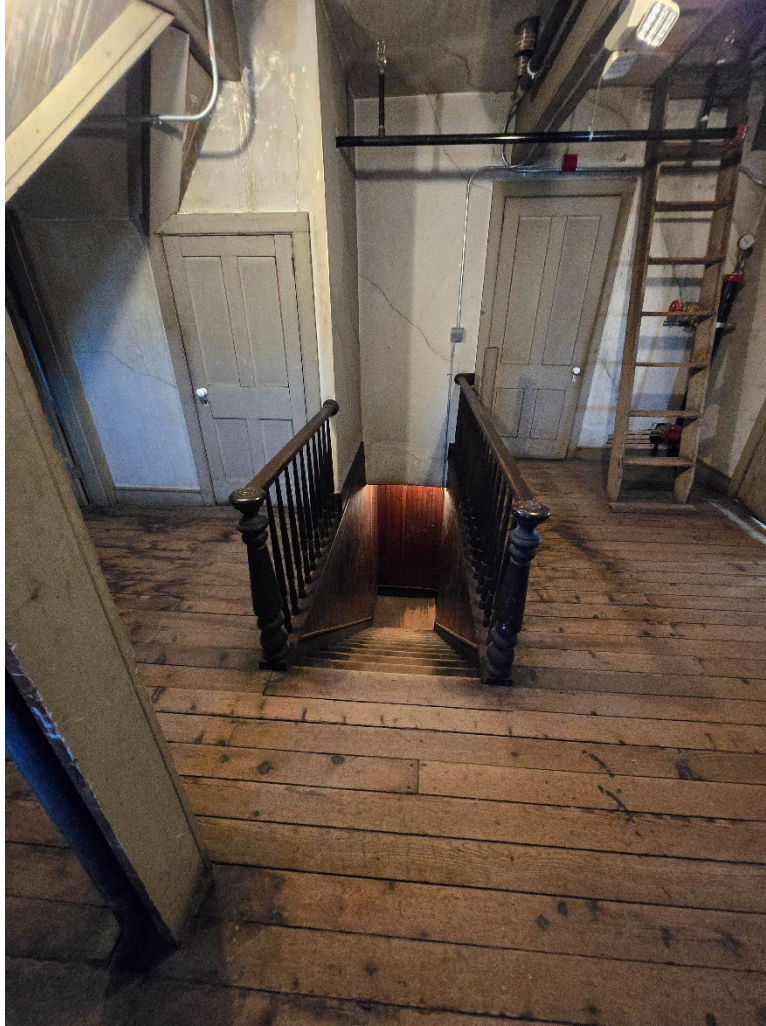
Photograph 61. Top of stairs leading to attic, view east.
