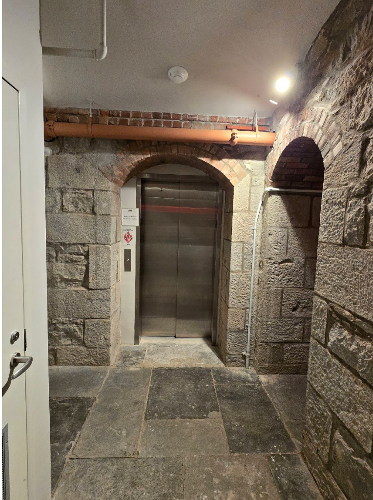
Photograph 68. Granite walls surrounding elevator shaft, view south.
