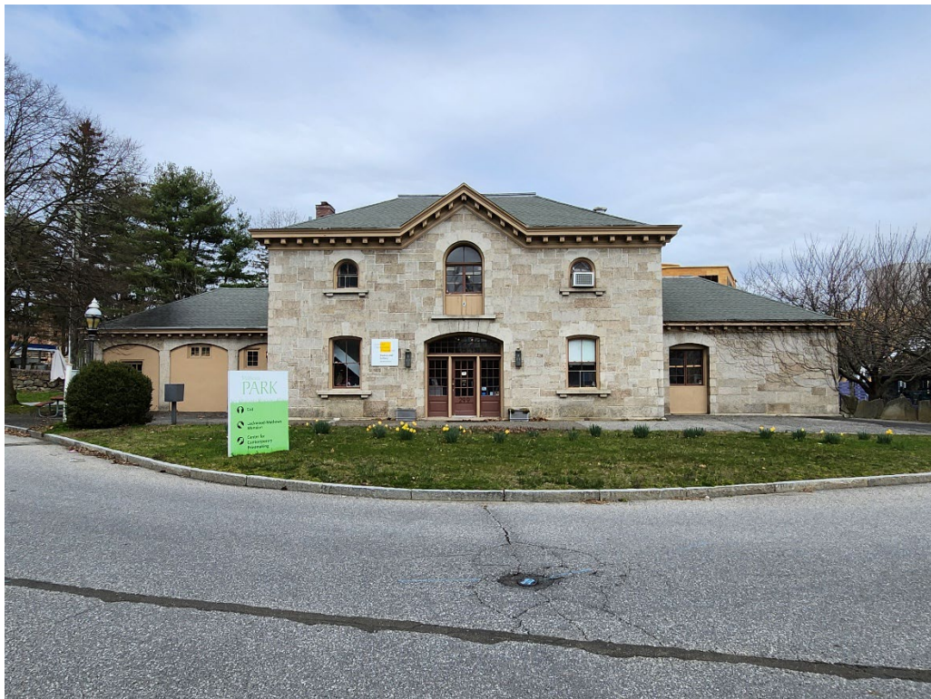
Photograph 85. Facade of Carriage House, view north.
