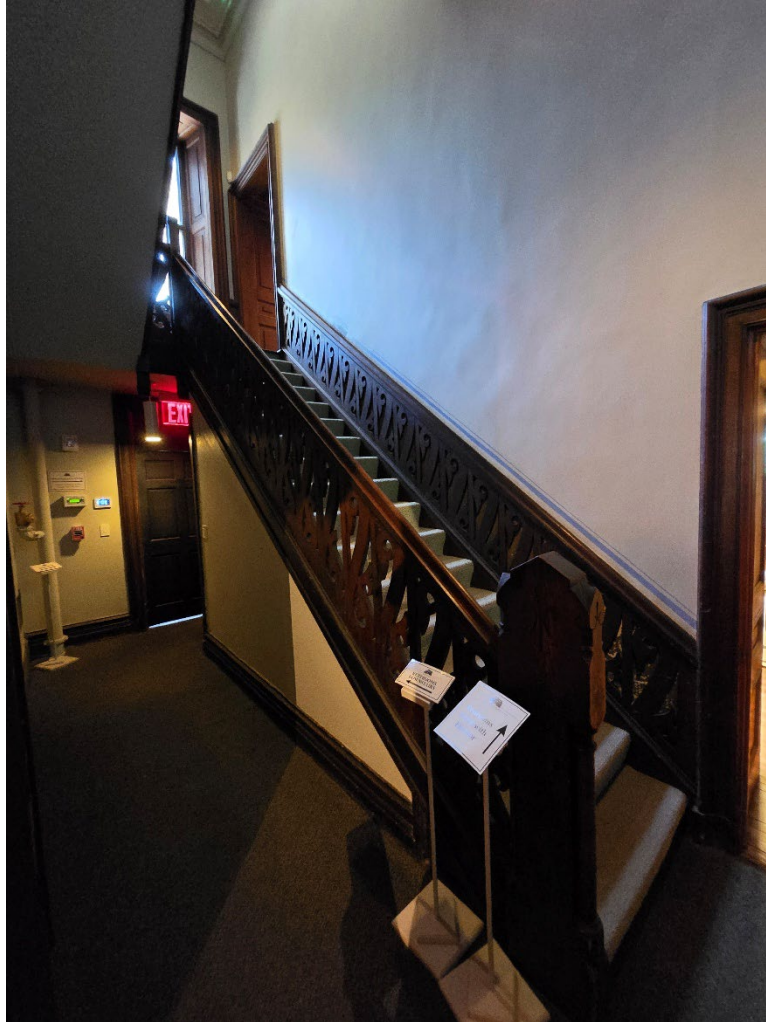
Photograph 16. Servants' staircase, flanking Grand Staircase, view northeast.
