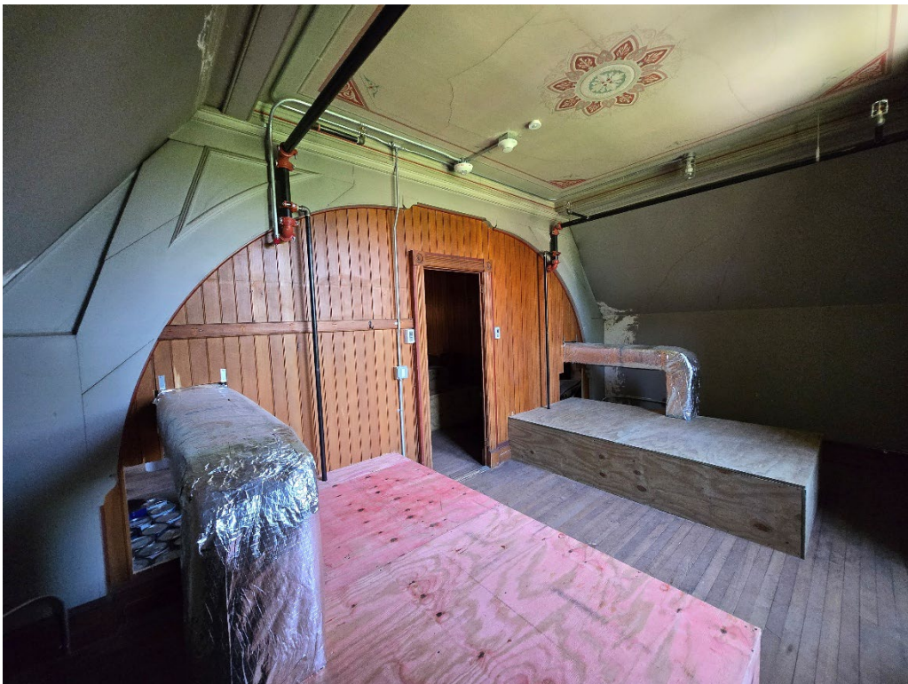
Photograph 58. Enclosed storage area on third floor, view southeast.
