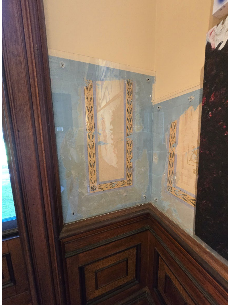
Photograph 31. Detail of original frescoes in Billiards Room, view northwest.
