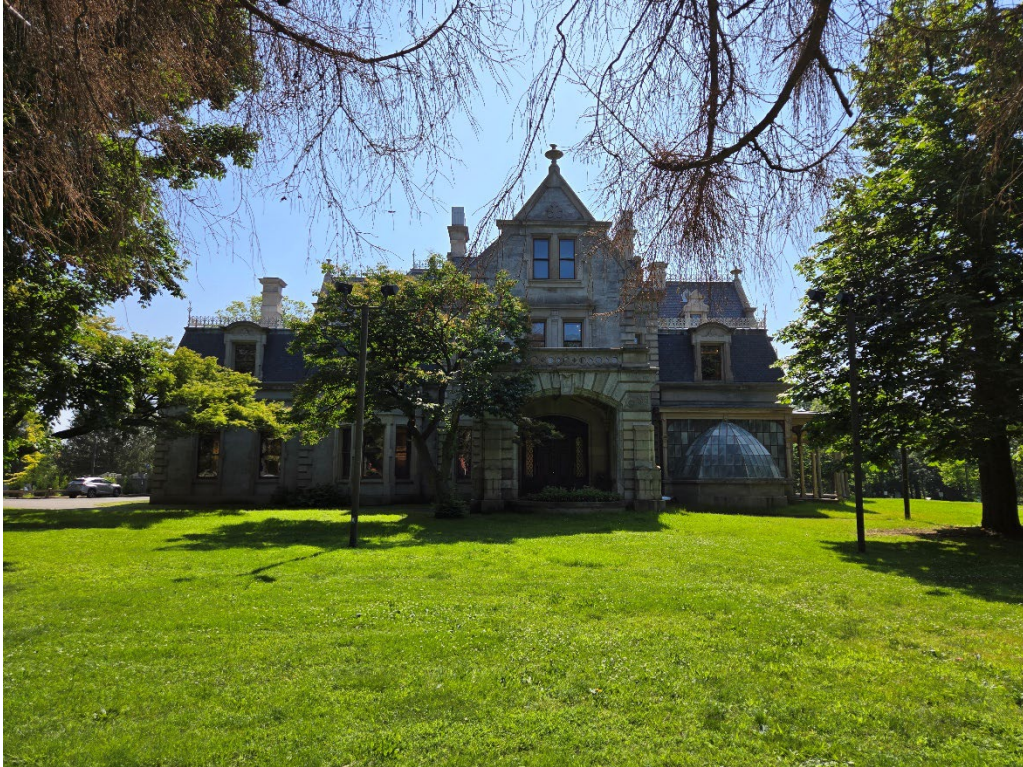
Photograph 3. Western elevation, view east.
