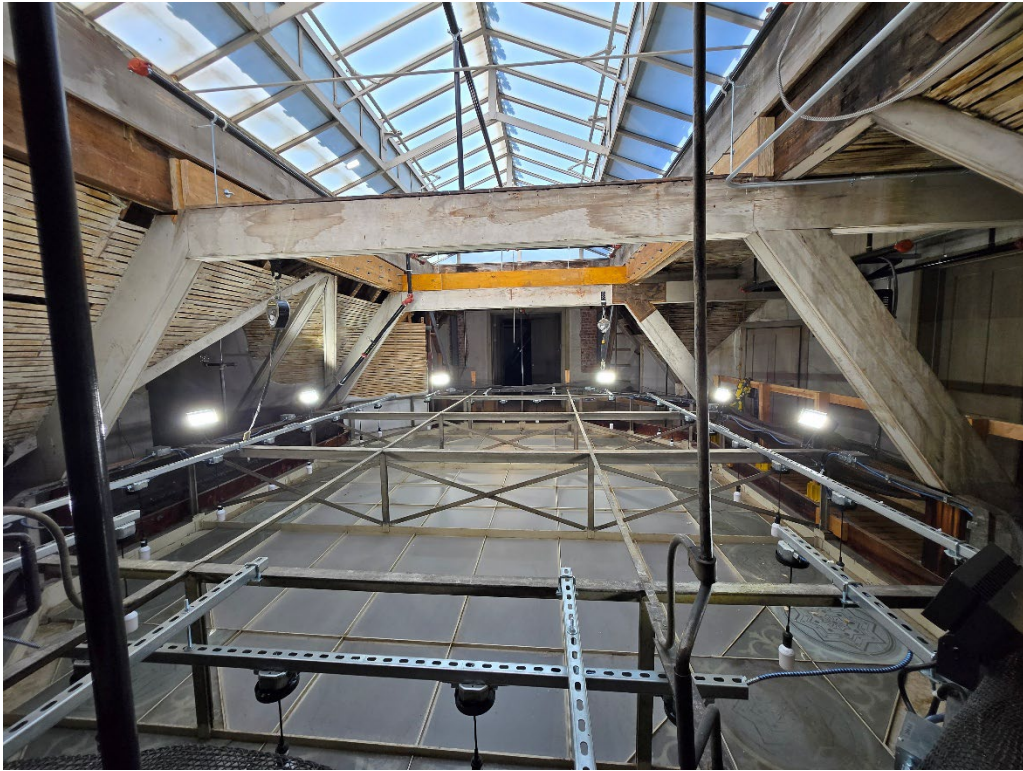
Photograph 62. Structural members in attic and skylight support, view west.
