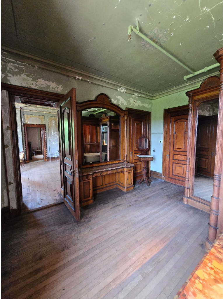
Photograph 46. LeGrand Lockwood's Bathroom, view west.
